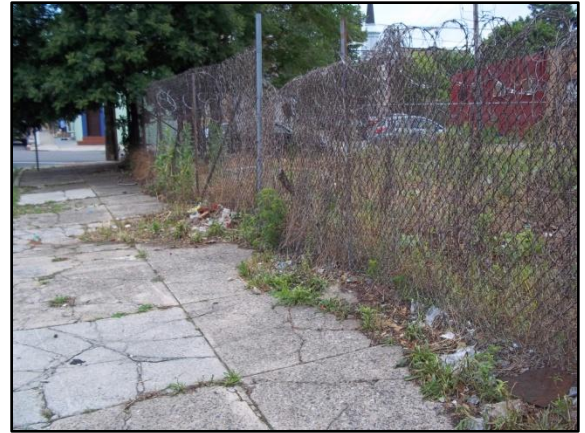
This fence surrounds a vacant property at Cadwallader and Oxford streets. The barbed wire is sagging, the fence is falling, and trash has collected along the back edge of the sidewalk. This is unsanitary and unsafe.
