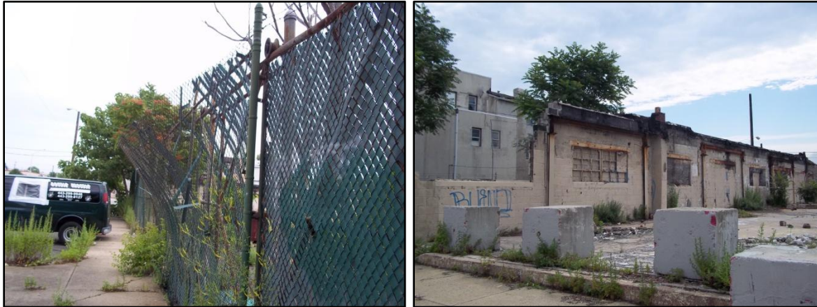
This fence (left photo) surrounds a vacant property on American between Oxford and Jefferson streets. The fence is leaning precariously into the right of way. Further north, this unsecured property (right photo) has attracted trash and graffiti. This is clear evidence of an unsafe and unsanitary condition. A side wall from the previous building barely stands next to an adjacent lot.
