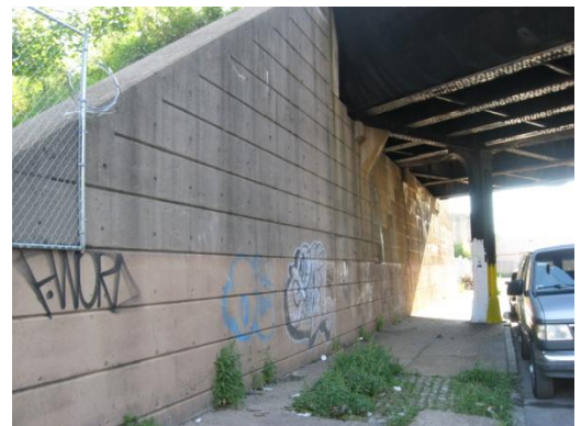
Reading Viaduct at Buttonwood Street
