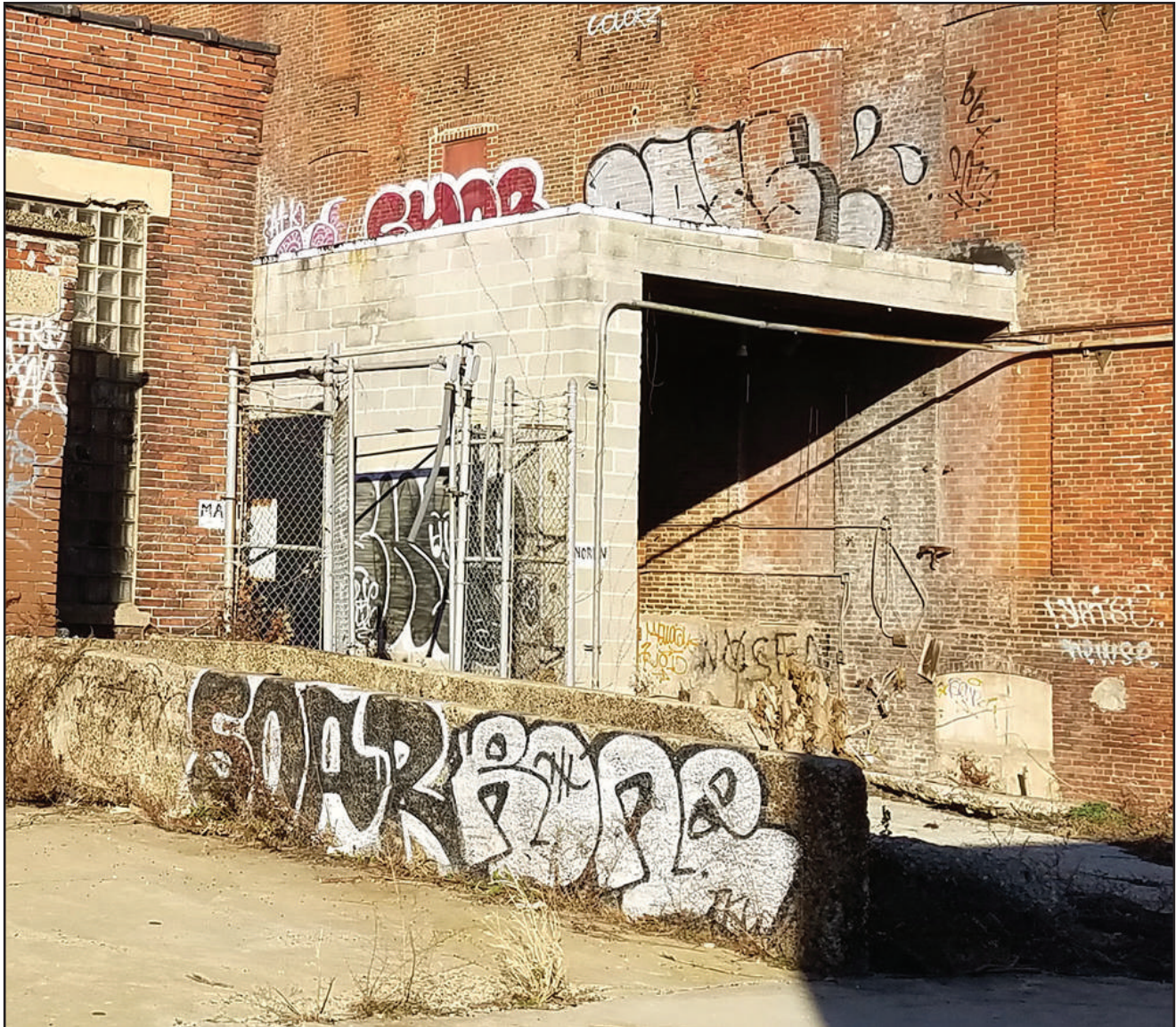
Figure 22: South elevation of the 1975 addition. | Photo: Dennis Carlisle
