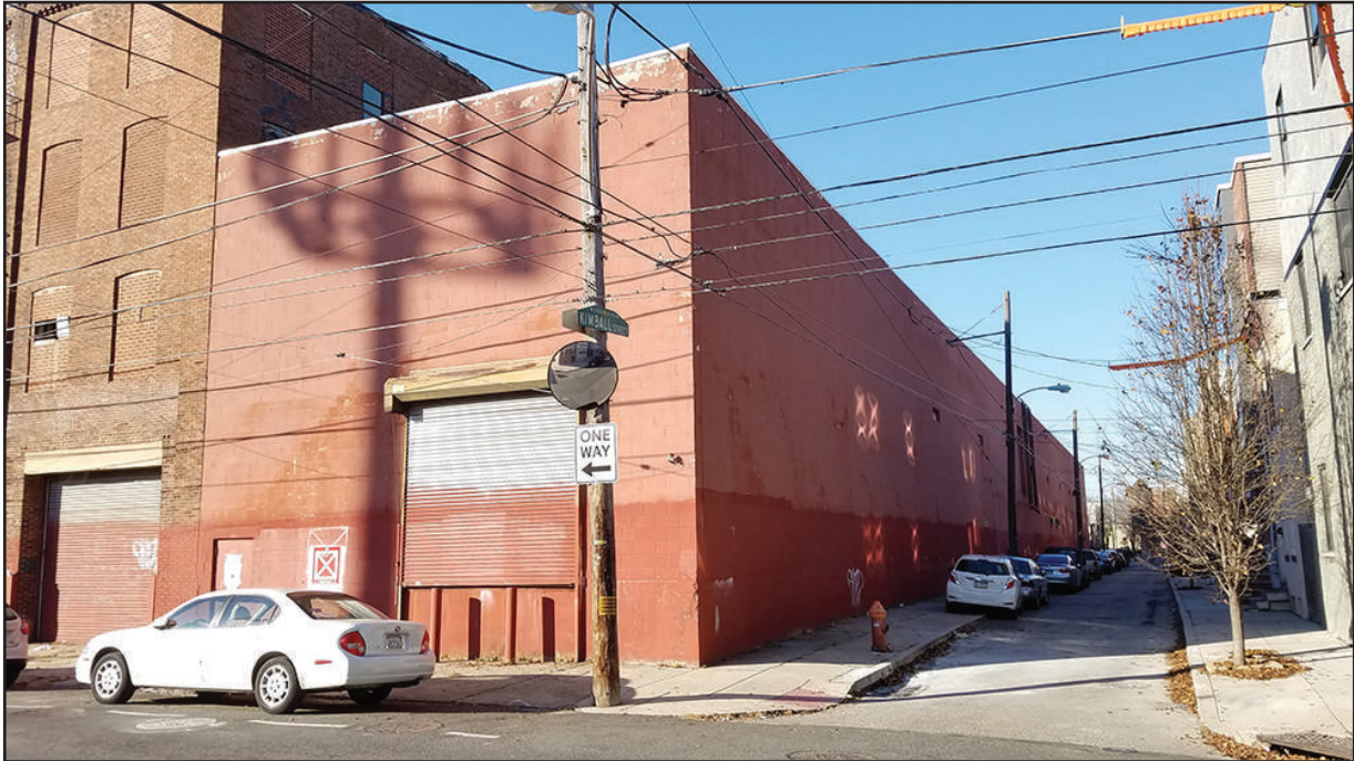
Figure 20: East and north elevations of the 1968 addition. | Photo: Dennis Carlisle
