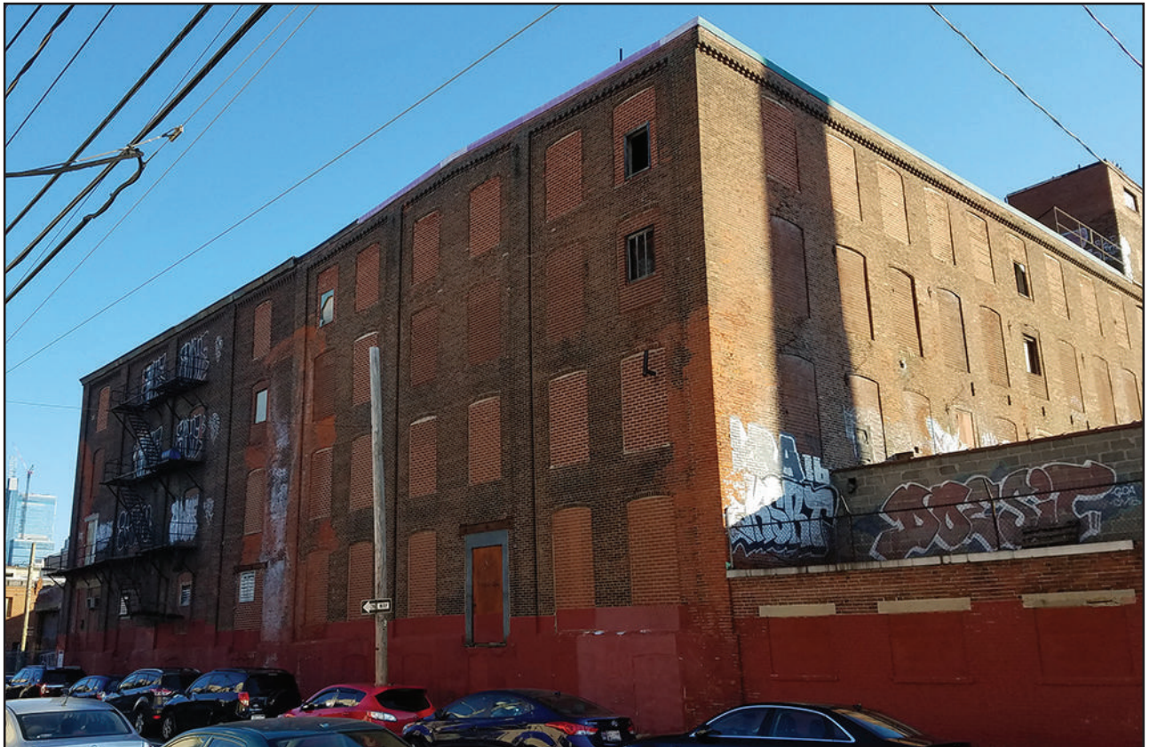
Figure 5: West elevation of the 1865 section. | Photo: Dennis Carlisle
