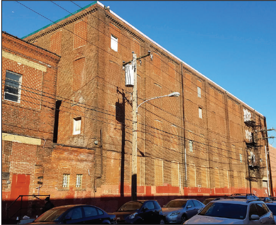
Figure 4: East elevation of the 1865 section. | Photo: Dennis Carlisle
