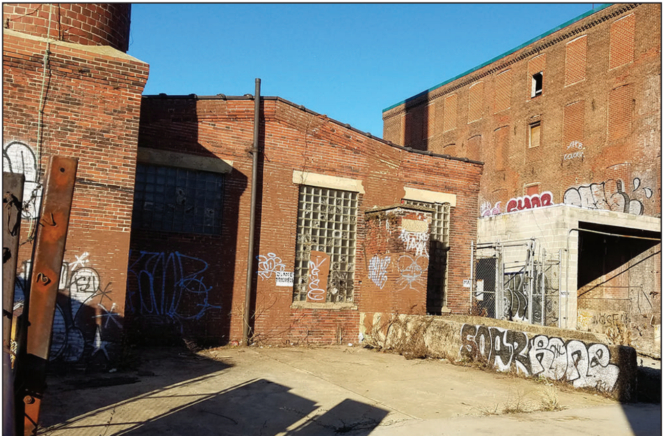
Figure 8: East elevation of the 1917 addition. | Photo: Dennis Carlisle
