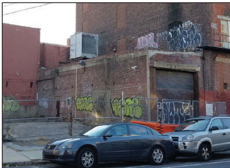
Figure 10: The only segment of 1912 Addition B visible from street level. | Photo: Dennis Carlisle
