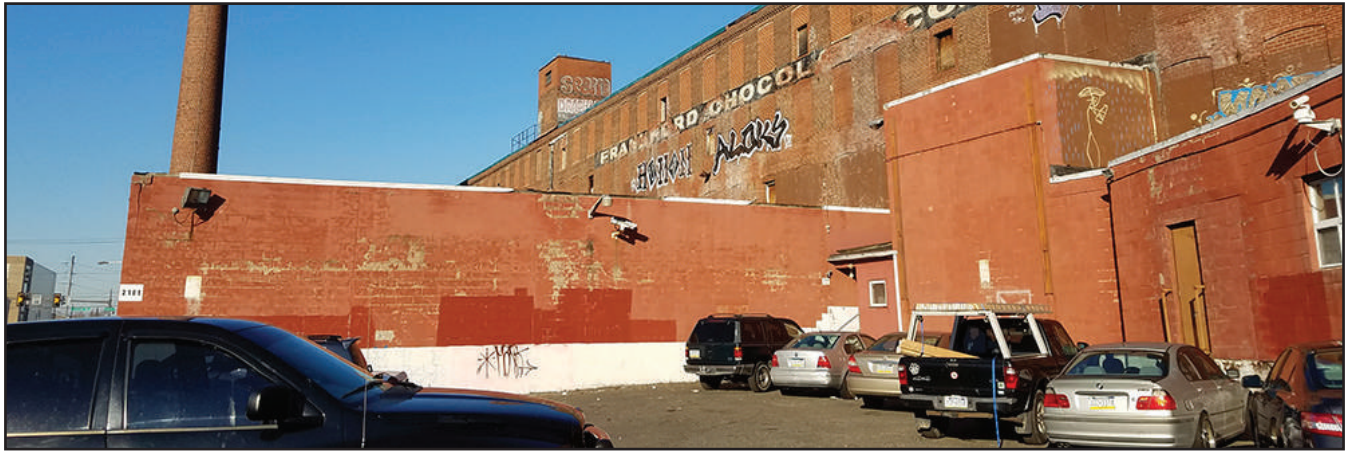
Figure 17: East elevation of 1967 Addition A with a portion of 1967 Addition B | Photo: Dennis Carlisle
