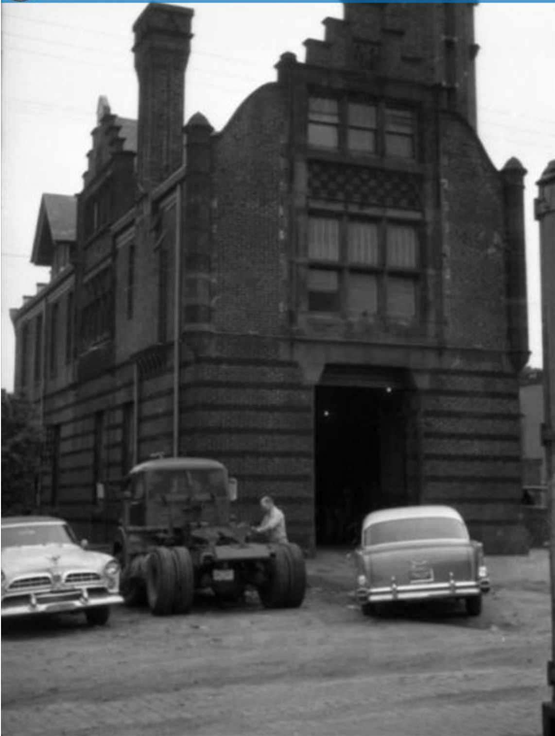
Figure 9: North and east elevations in 1963. DOR archive photo, http://www.phillyhistory.org/photoarchive/Detail.aspx?assetId=86586
