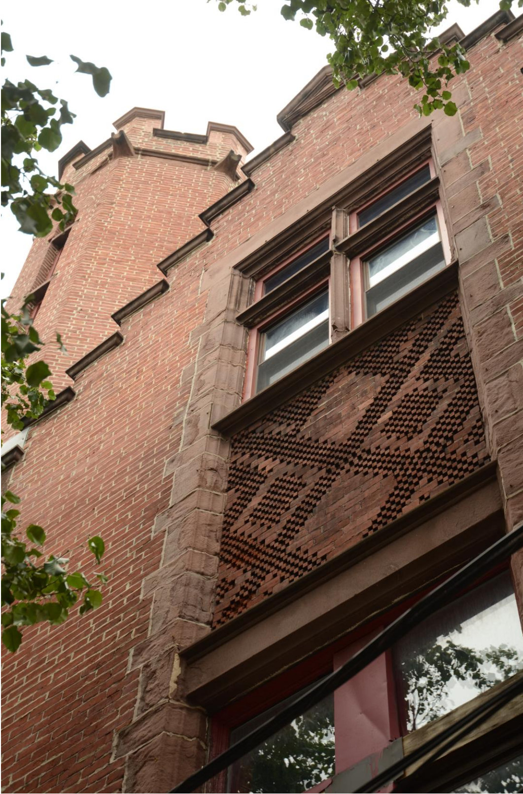
Figure 7: West (Water Street) elevation detail of corner tower, cross-gable and textured brick spandrel.
