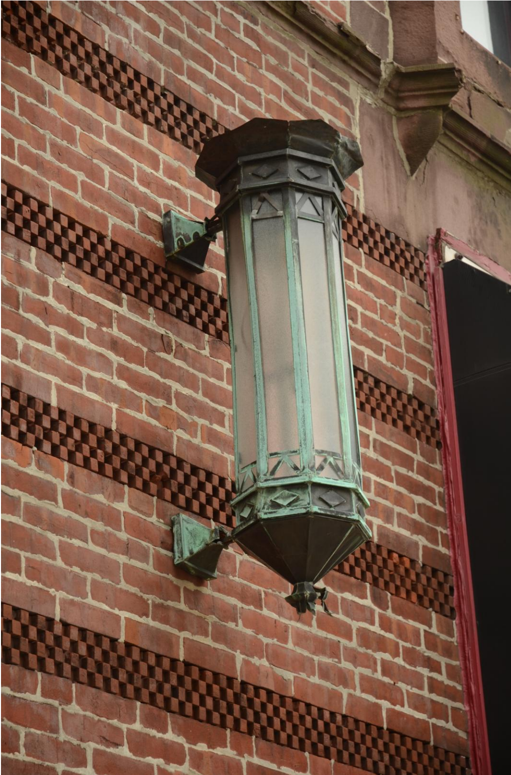
Figure 6: North elevation detail of sconce and textured brick courses. The scones, while historic fixtures, do not appear to be original to the building (see Figures 8 and 9).
