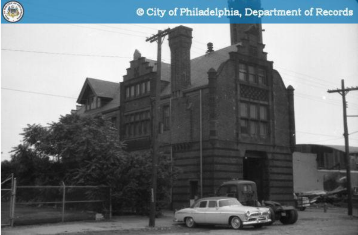
Figure 10: North and east elevations in 1963. DOR archive photo, http://www.phillyhistory.org/photoarchive/Detail.aspx?assetId=86587
