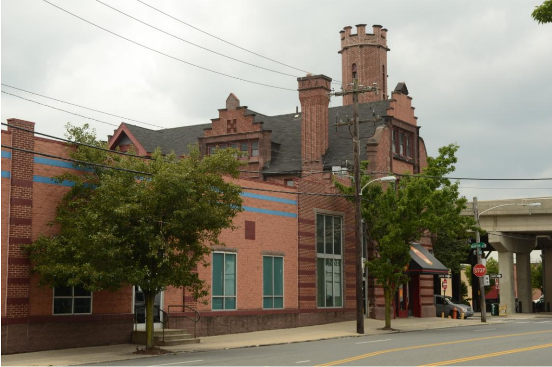
Figure 3: Site view facing southwest, showing north and partial east elevations. The majority of the foreground addition stands on a separate parcel from the historic firehouse and is not subject to this nomination.
