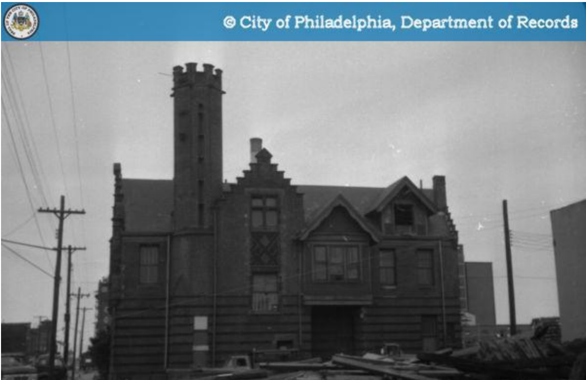
Figure 11: West elevation in 1961. DOR archive photo, http://www.phillyhistory.org/photoarchive/Detail.aspx?assetId=86584
