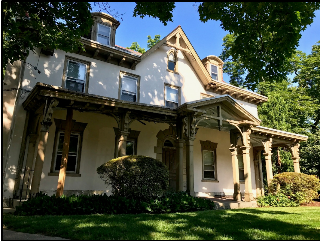
Looking west at the Primary Elevation of the Main block. Source: Brad Maule.
