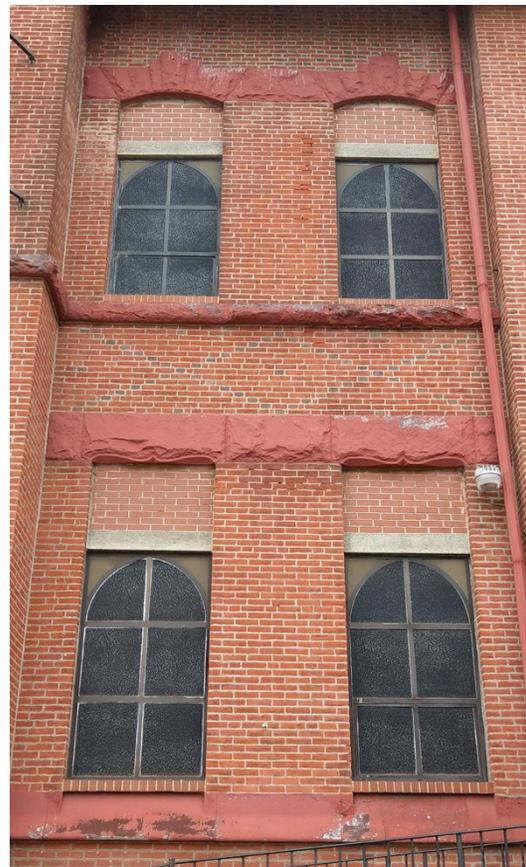
Figure 2: South elevation detail showing chamfered lintels and diamond brick patterning.
