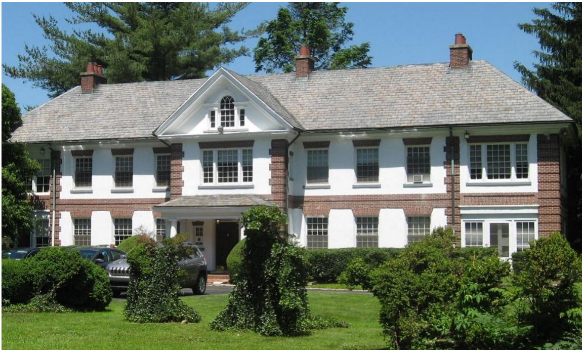
Figure 13: Current photograph. When compared to the historic photograph of the property, it is clear that the building retains nearly all of its original features.
