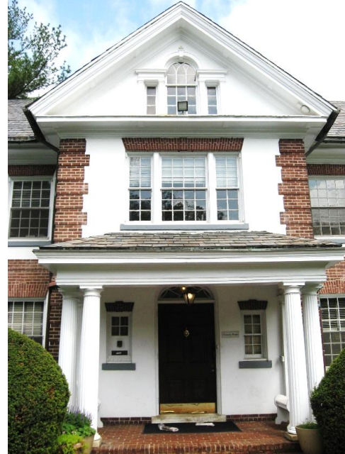
Figure 5: Central projecting bay.
