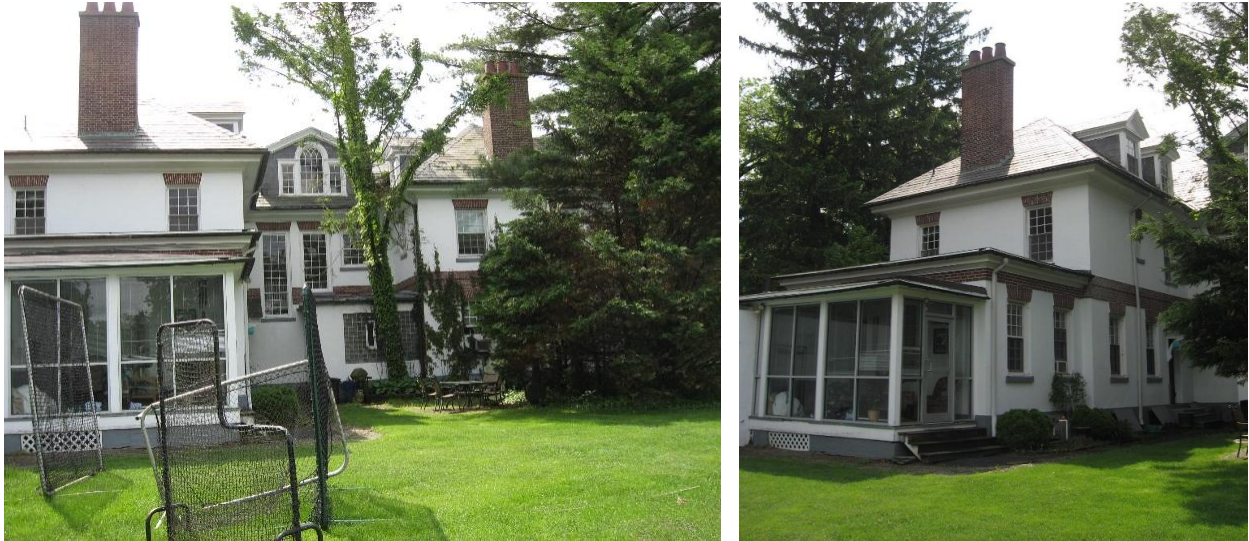
Figure 8: (Left) North elevation with east extension; (Right) Larger, east, rear extension.
