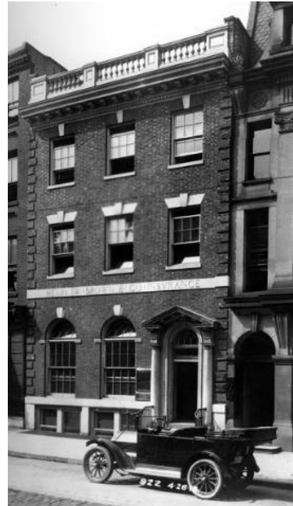
Figure 17: 1915 photograph of Henry W. Brown & Co. office building (1910), 433 Walnut Street. One of the last designs by Clinton Gardener Harris, who died the same year. This block of Walnut Street was demolished in the 1950s for Independence Mall. Source: Philadelphia Historical Commission.
