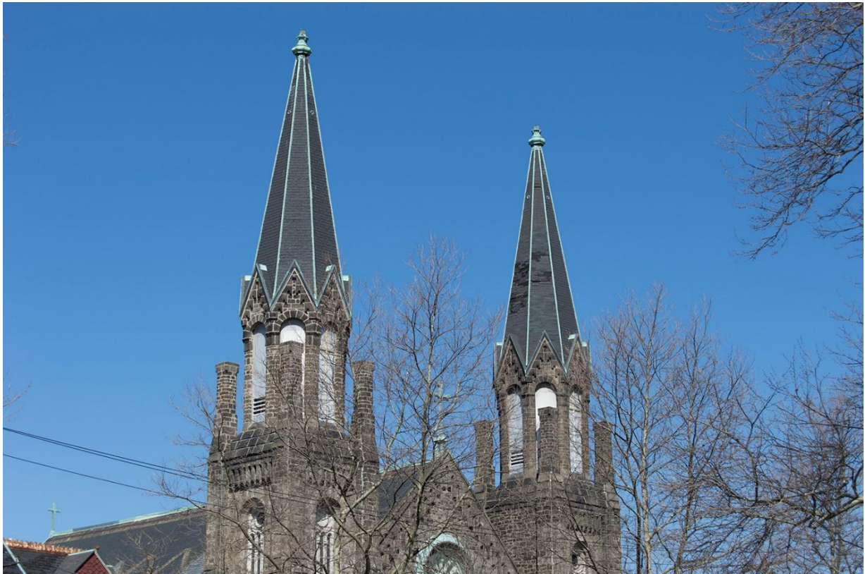
Figure 3: Towers of Our Mother of Sorrows Catholic Church at 48th Street and Lancaster Avenue. 2015.
