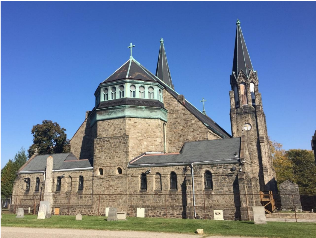
Figure 6: West (rear) facade featuring octagonal apse and distinct apse windows. 2015.
