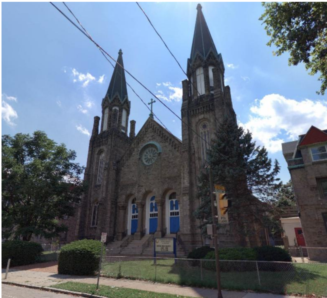
Figure 1: Front (east) elevation of Our Mother of Sorrows. Source: Cyclomedia, 2017.
