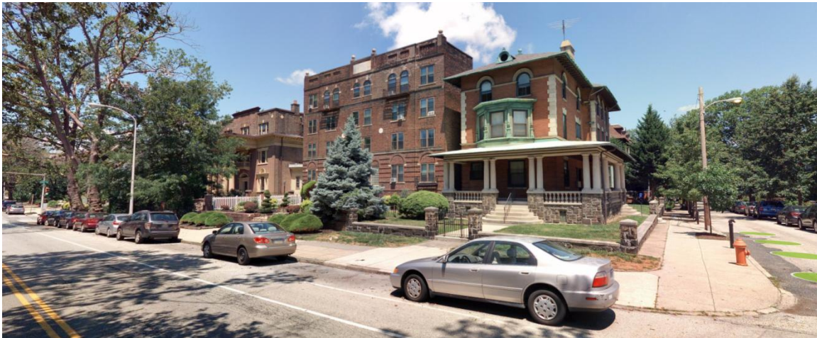
Figure 3. 4525 Spruce Street, shown with its neighbors at 4529-33 and 4537 Spruce Street. Source: CycloMedia, 7/2/2017.
