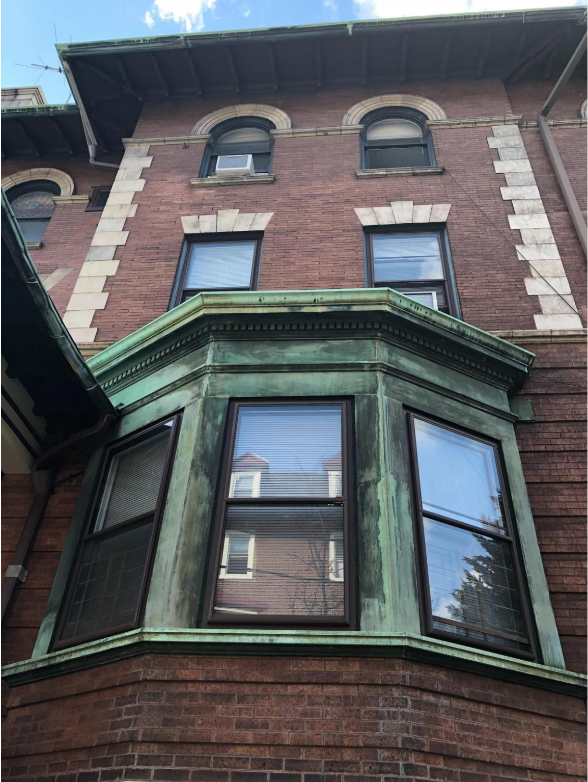
Figure 12. Bay detail on Melville Street side. Source: Corey Loftus.
