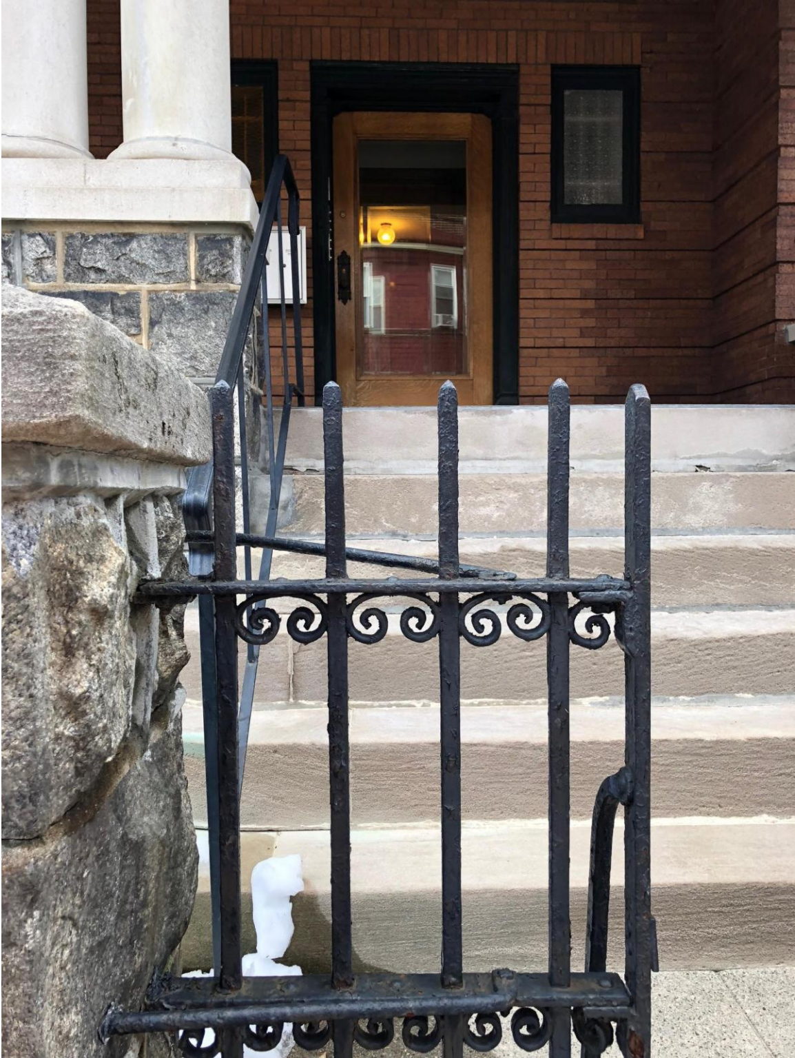
Figure 13. Iron gate at front entrance on Spruce Street. Source: Corey Loftus.
