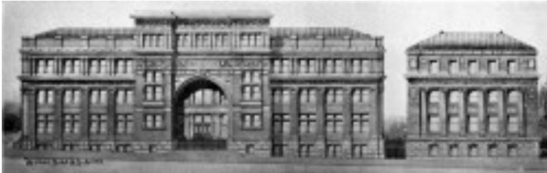
Figure 6. The Drexel Institute of Technology (main building) 3101 Chestnut Street. Builder: Charles McCaul. Source: King, Moses. Philadelphia and Notable Philadelphia . (New York: Blanchard Press, Isaac H. Blanchard Co., 1901), p. 24d.
