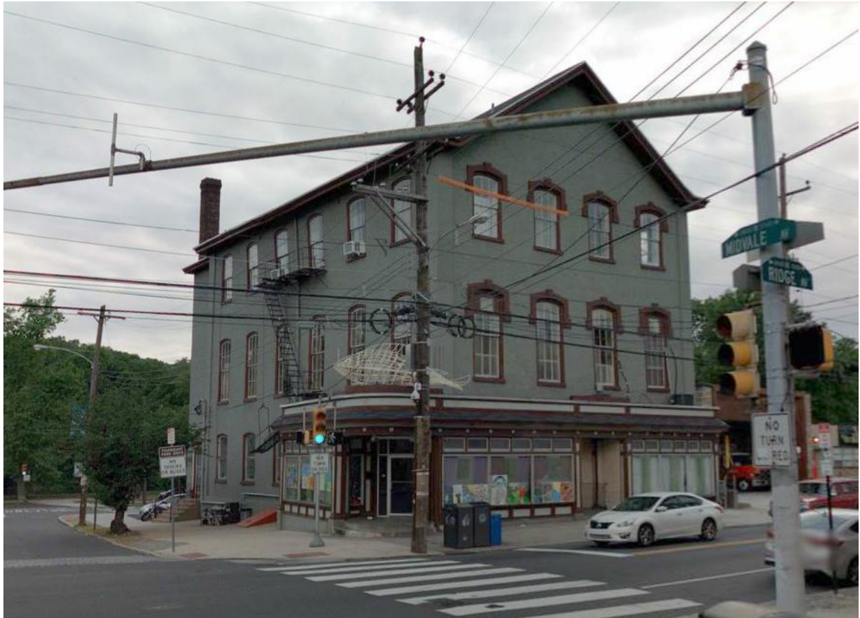
Figure 4: Oblique view of the former Odd Fellows' Hall, situated at the intersection of Ridge and Midvale Avenues (all photographs from Cyclomedia, August 2017, unless otherwise noted).
