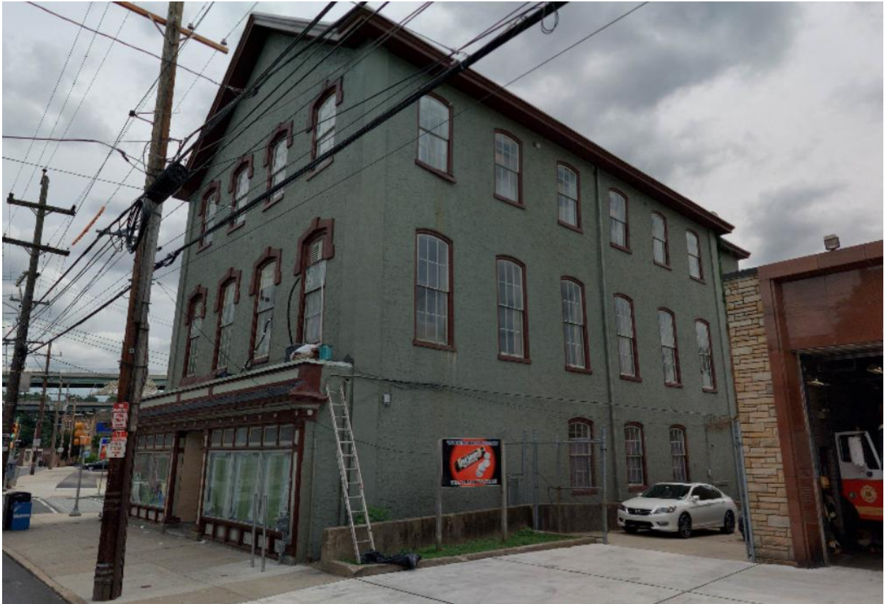
Figure 12: West elevation, as visible from Ridge Avenue.
