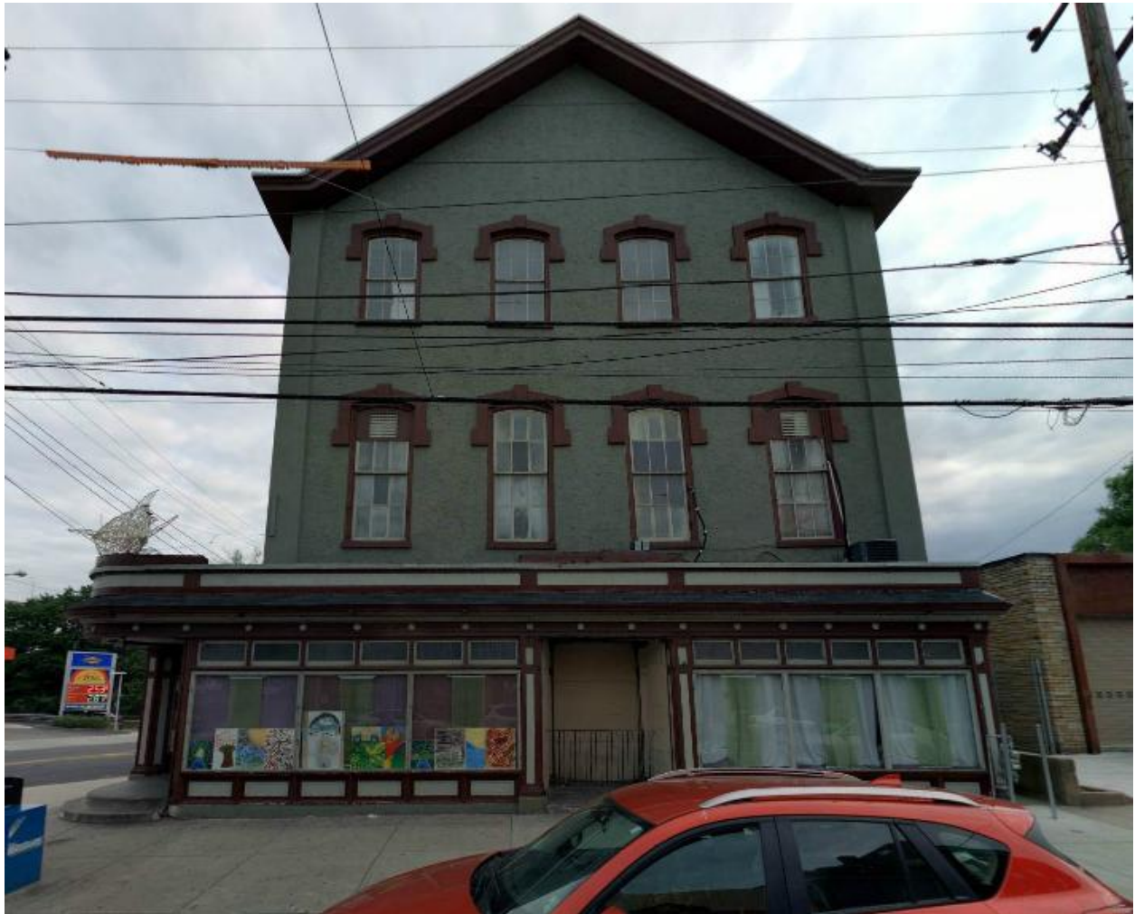
Figure 7: The primary, north, elevation faces Ridge Avenue.
