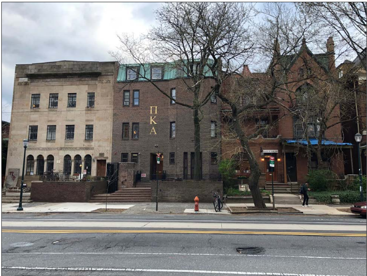
Photograph of 3912-3922 Spruce Street. 3920 Spruce Street is the third property from the left. Constructed in 1890, the building was developed by William Weightman and designed by Willis Hale. All buildings were originally designed by Hale but 3912-14 Spruce Street and 3916-18 Spruce Street have undergone significant alteration, rendering them unrecognizable from their original design. Photograph courtesy Corey Loftus.
