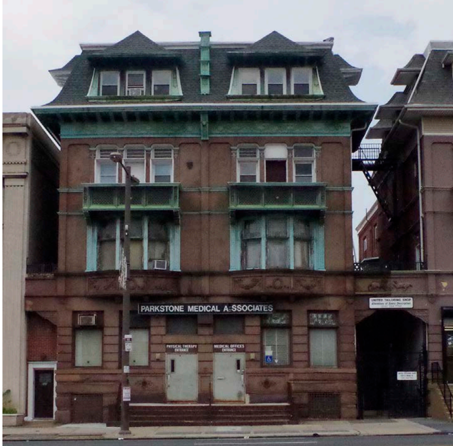
Front elevation of 2305-07 N. Broad Street. Photo: Author.
