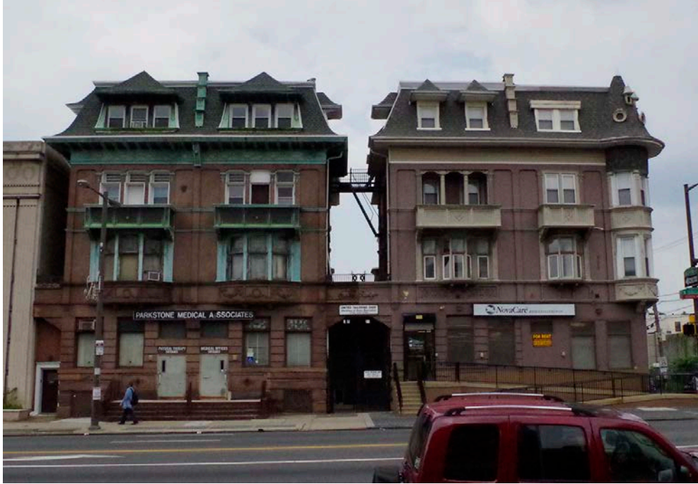
The facades of 2301-07 North Broad Street, connected by a brownstone arch formed from the belt course supporting the oriel windows of the piano nobile at each dwelling. Photo: Author.
