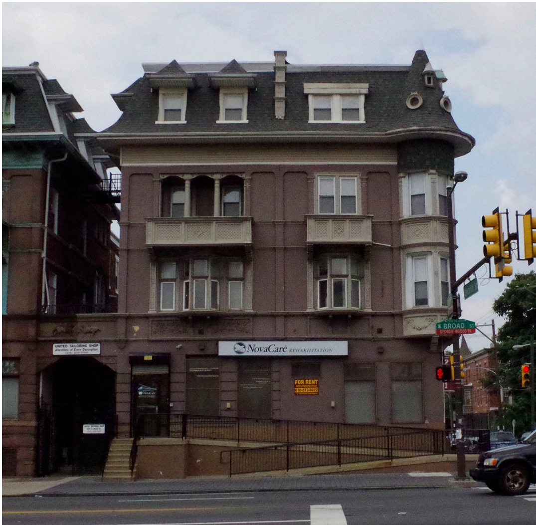
West elevation and façade of 2301-03 North Broad Street.
