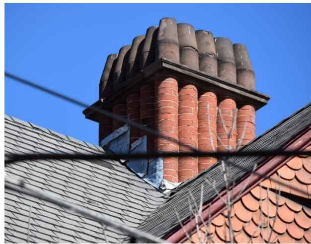
Figure 10: Chimney stack with molded brick. Looking northeast.
