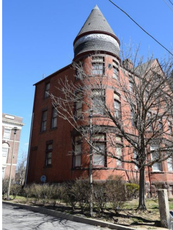
Figure 12: Southwest corner of building viewed from Parrish Street. Facing northeast.
