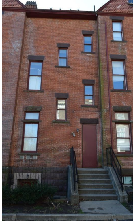
Figure 15: Central bays of north elevation with diagonal fenestration. Looking south.
