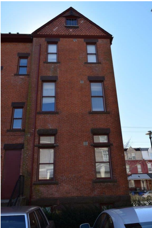
Figure 16: Westernmost bays of north elevation. Looking south.
