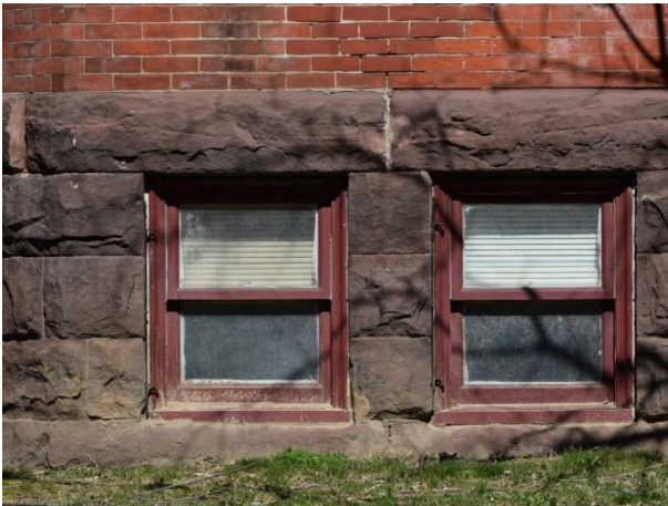
Figure 2: Rusticated brownstone water table with typical fenestration at base of building.
