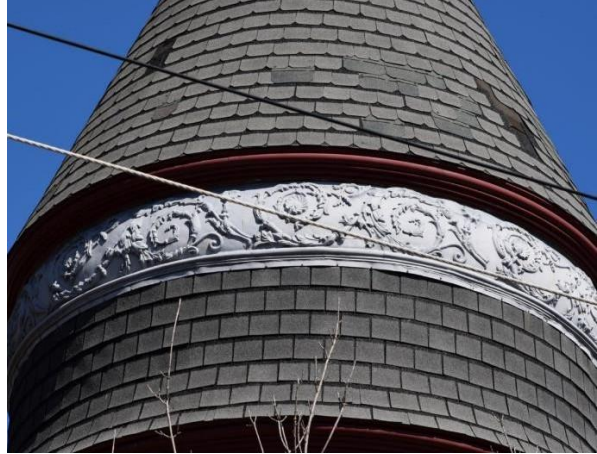
Figure 6: Detail of shingles and decorative band found on both turrets.
