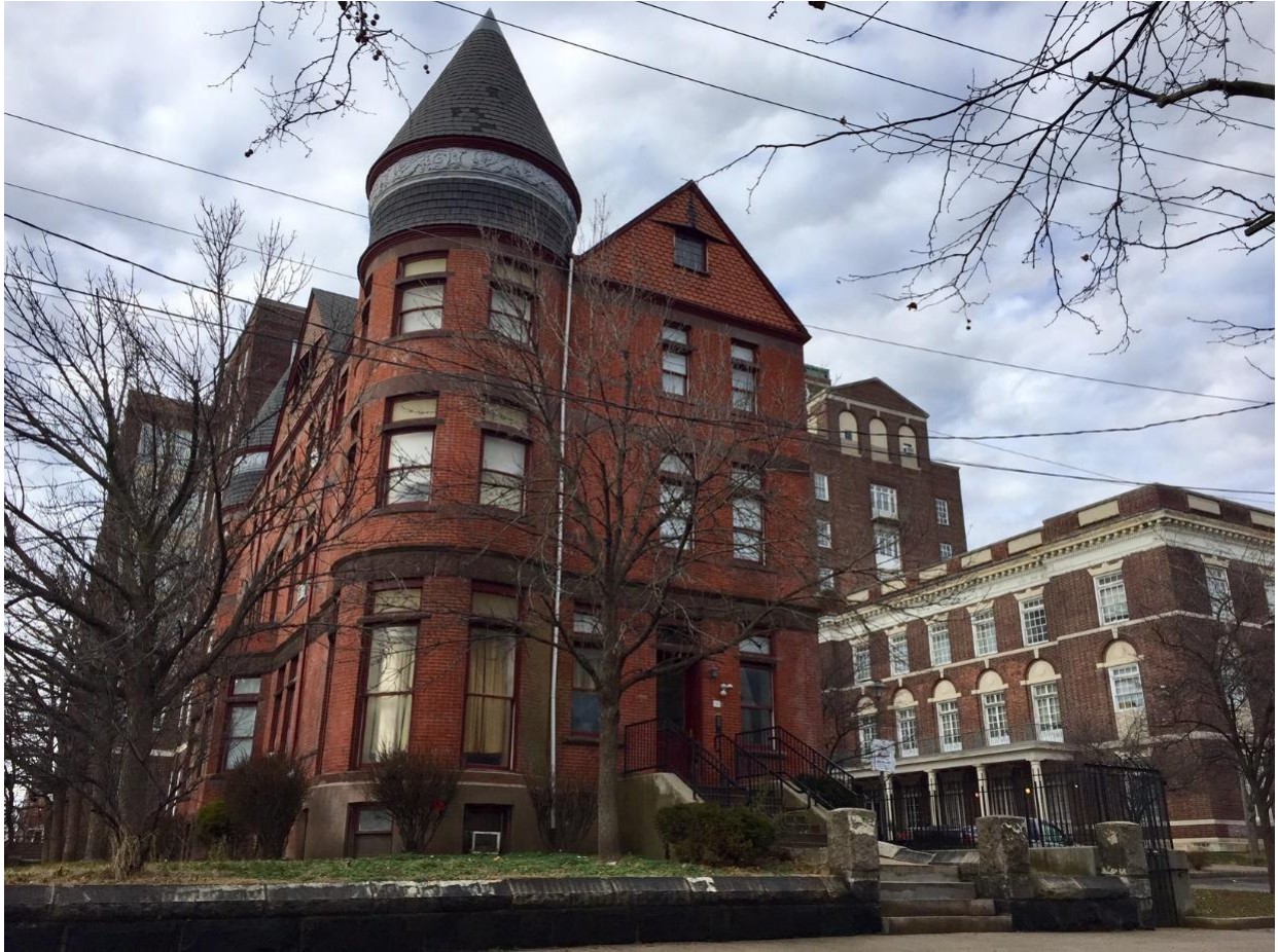
Figure 4: East elevation viewed from N. Preston Street.
