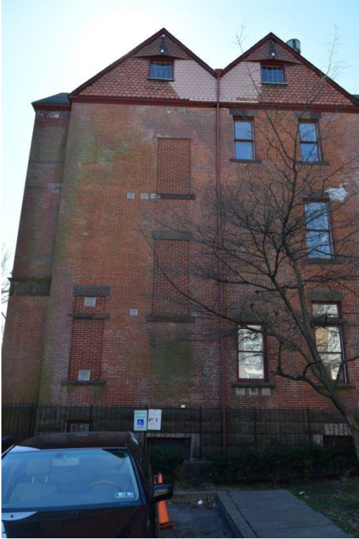
Figure 14: Easternmost bays of north elevation. Looking south.
