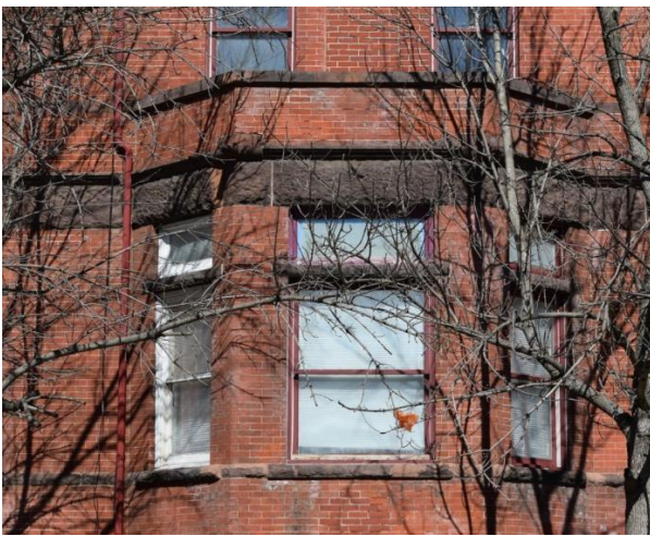
Figure 9: Projecting bay window at first floor, south elevation. Looking north.
