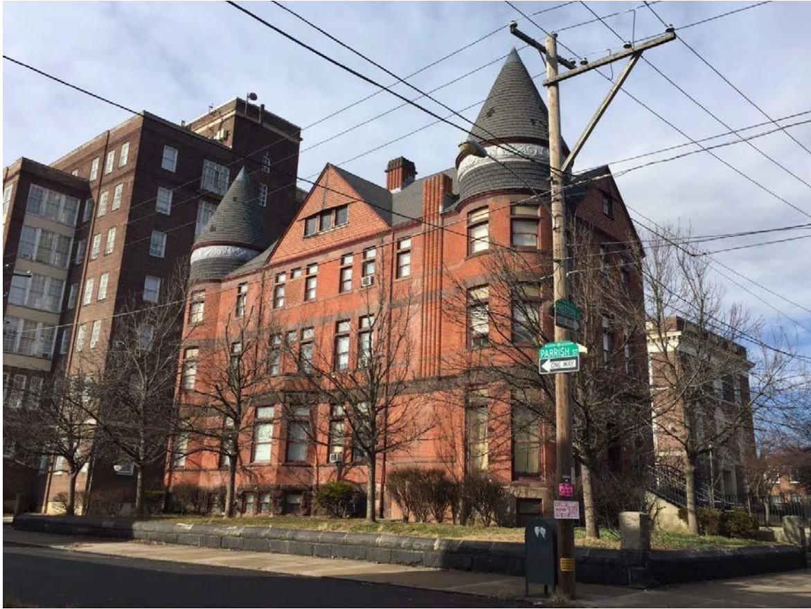
Figure 1: 836 N. Preston Street viewed from intersection of N. Preston and Parrish streets, January 2017. Facing northwest.
