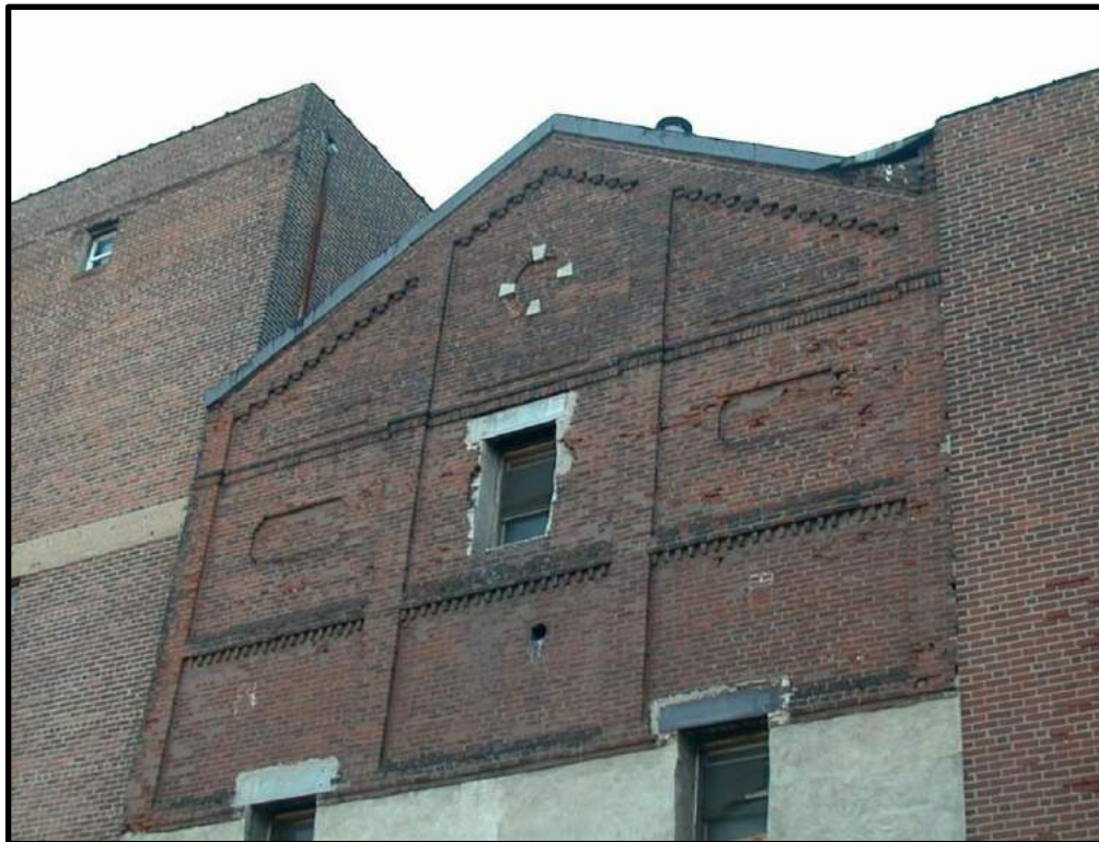
Figure 30. Looking west, above is the rear view of Building No. 2. While the primary elevation of this late nineteenth century building has been modernized, the rear elevation features original details at the top floors. Source: Richard Wagner, Pennsylvania Brewery Historian.
