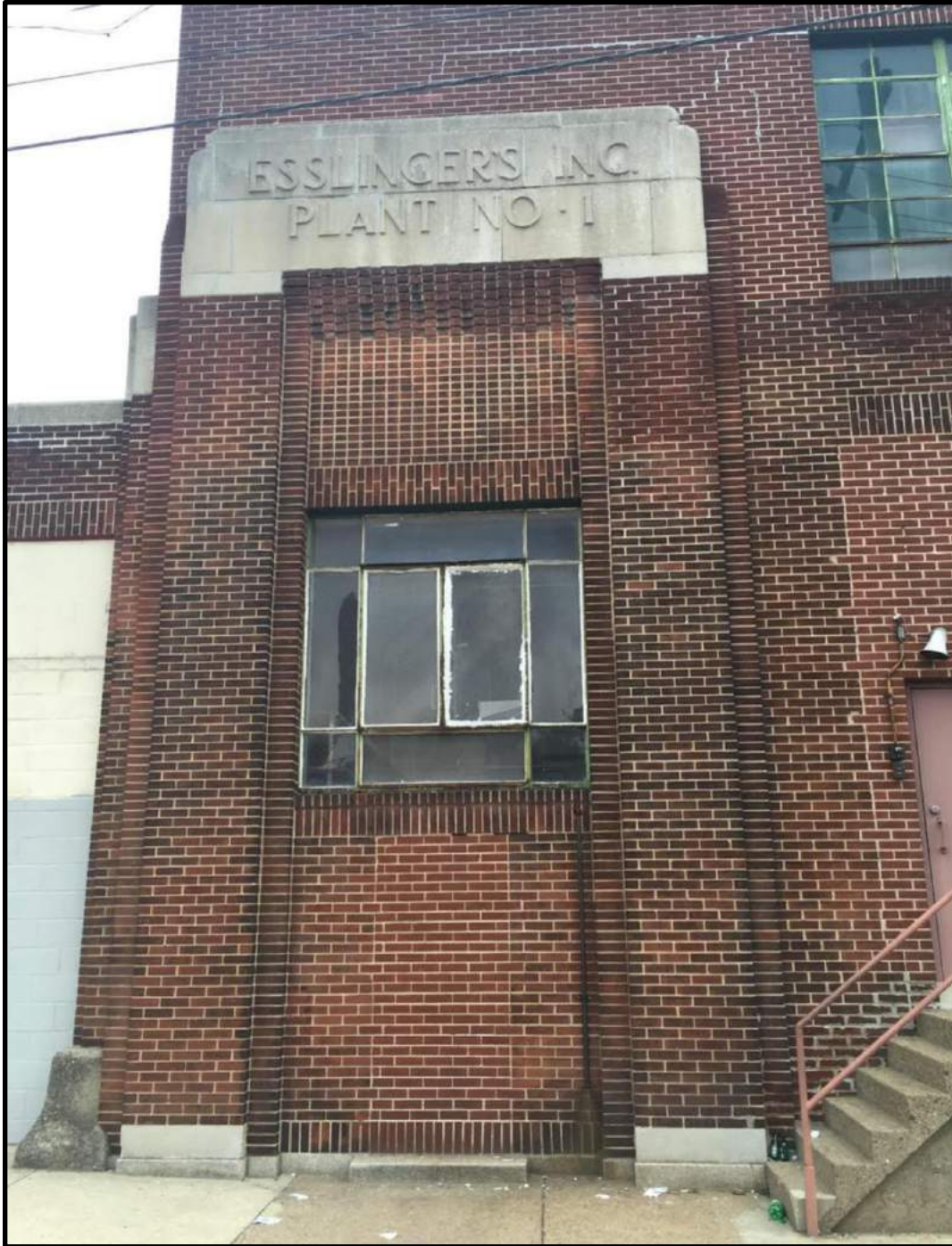
Figure 17. Looking east, the brick and stone details of Building No. 8C of Building No. 8. This image further depicts the brick pilasters with stone capitals, etc. with the raised lettering, “Esslinger’s Inc., Plant No. 1” all of which is featuring traditional forms in the Modernist style. Source: Oscar Beisert.
