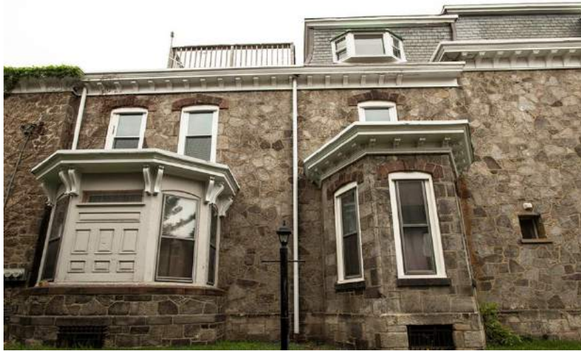
Figure 14: West façade of Rear Ell.
