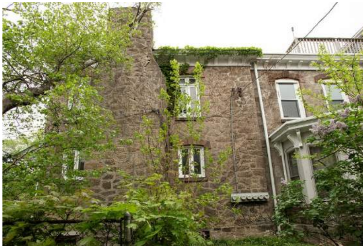
Figure 15: West façade of the Rear Addition.
