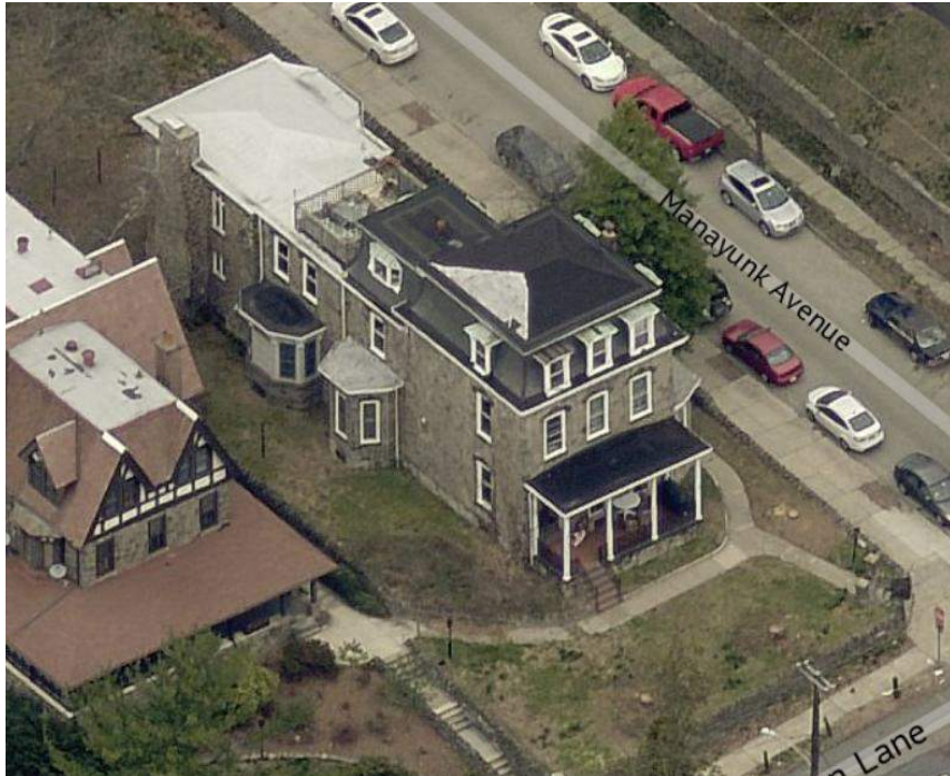
Figure 12: Aerial View of the West façade, looking north. Source: Pictometry.
