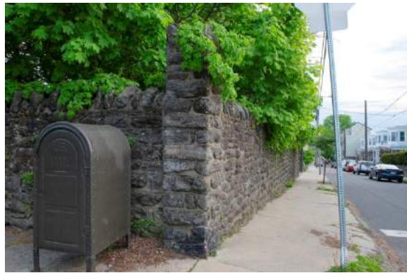
North-facing wall along Dupont Street.
