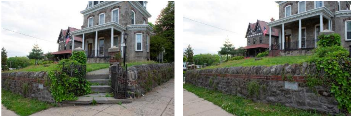
Figure 16: Southeast corner entrance steps and south-facing retaining wall with name plaque.
