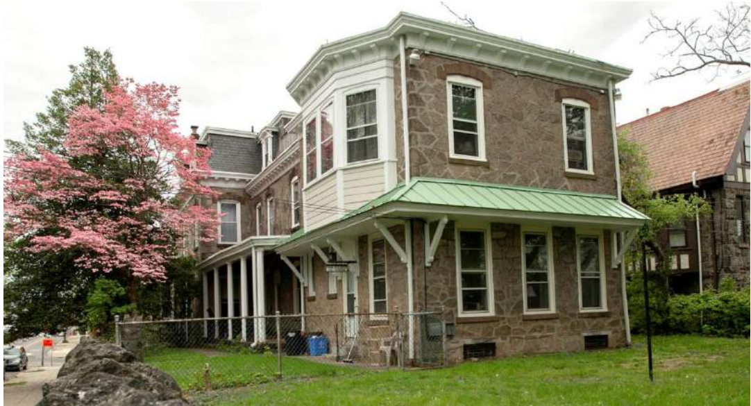
Figure 8: The north façade of the rear addition.
