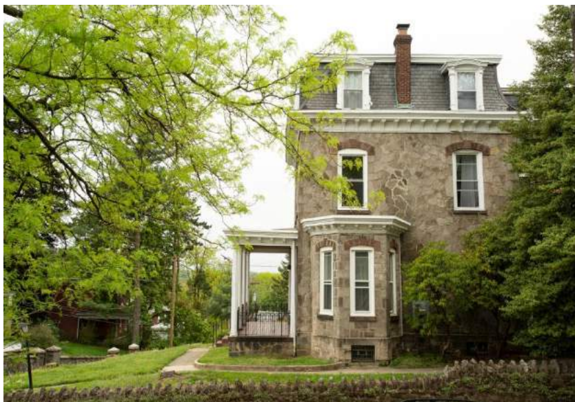
Figure 5: East elevation of the main block.
