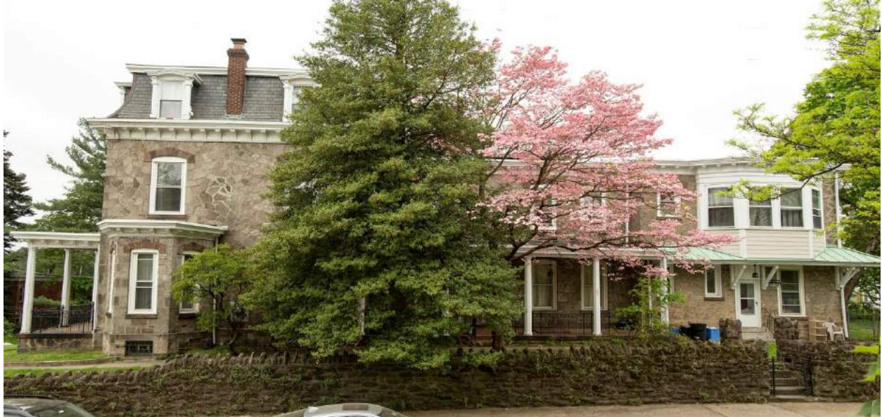
Figure 4: East façade, which is divided into three sections.
