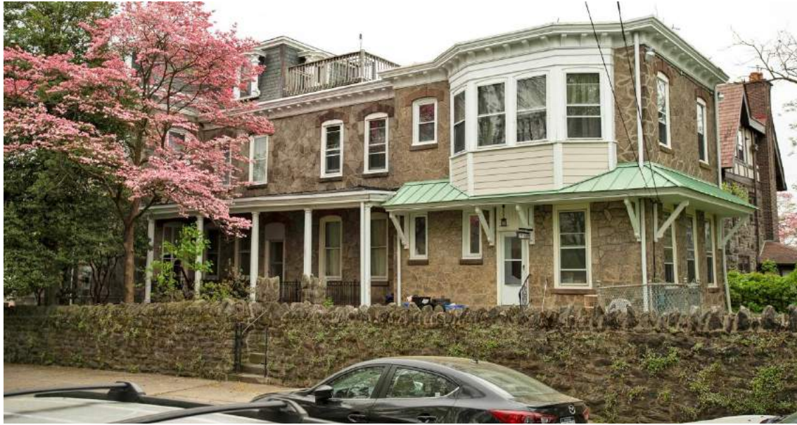
Figure 6: The central and rear side sections of the East Façade.
