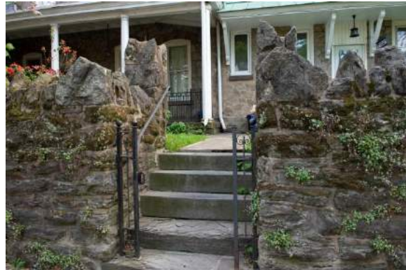
Steps on East-facing wall, Manayunk Avenue
