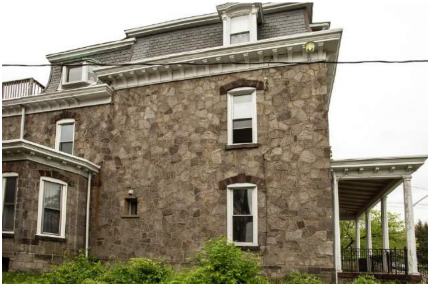
Figure 13: West façade of the Main Block.
