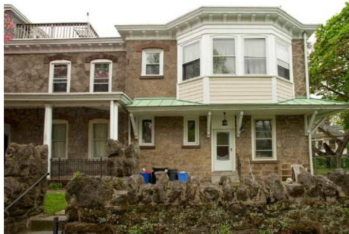
Figure 7: The east elevation of the rear addition.
