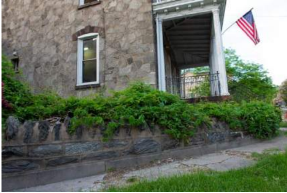
Southwest corner as wall wraps to front
