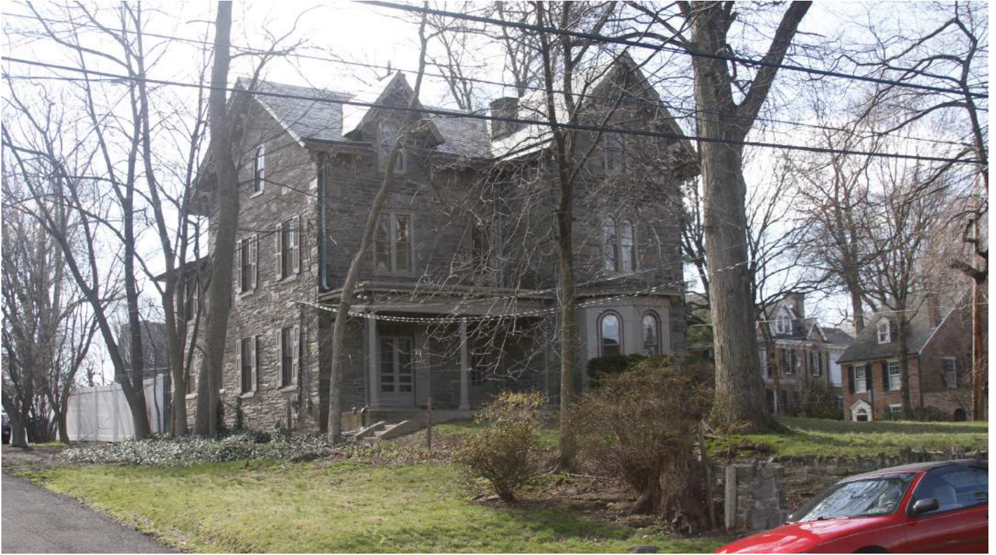
3. Northwest and northeast elevations, looking south from E. Chestnut Hill Ave.
