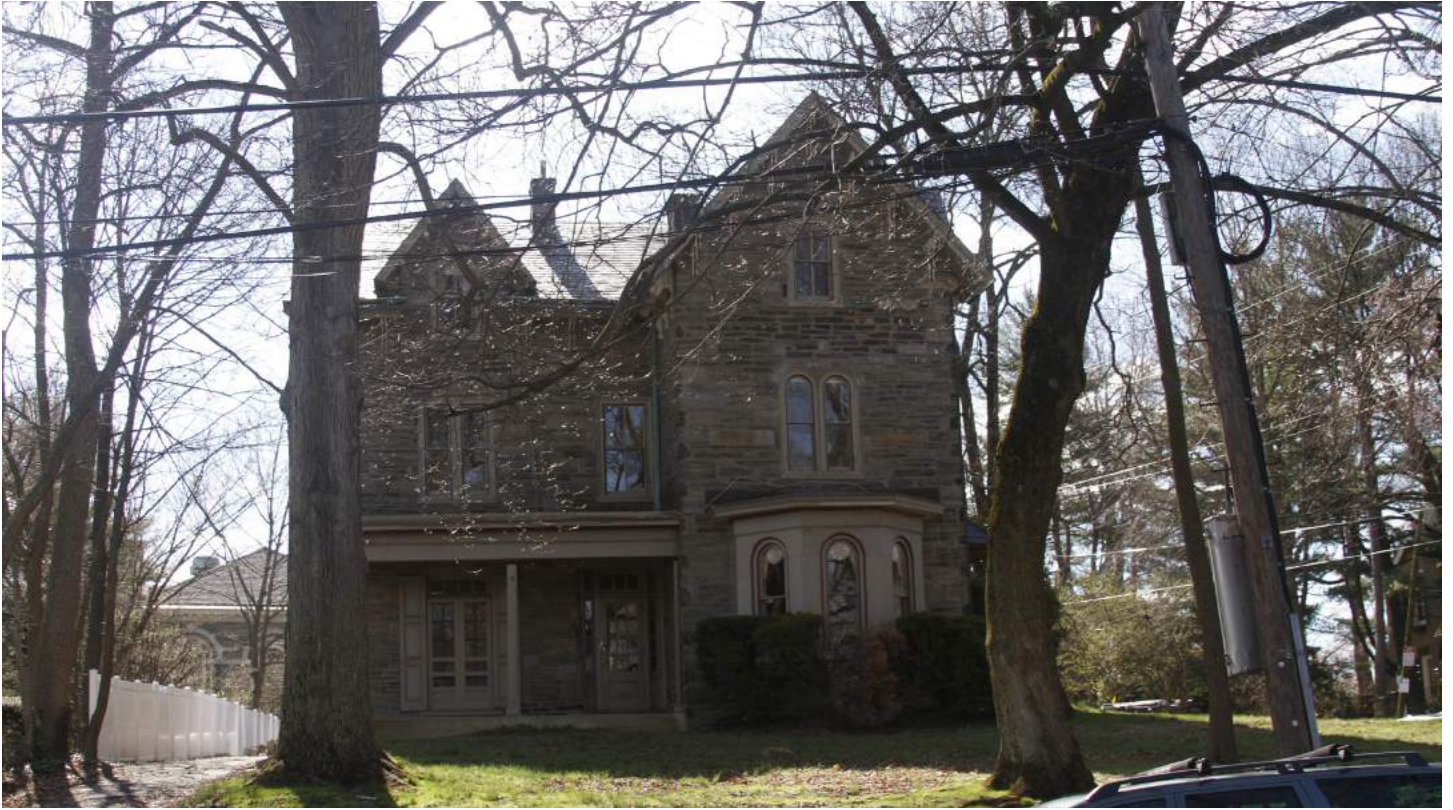
1. Northwest elevation, looking southeast from E. Chestnut Hill Ave.
