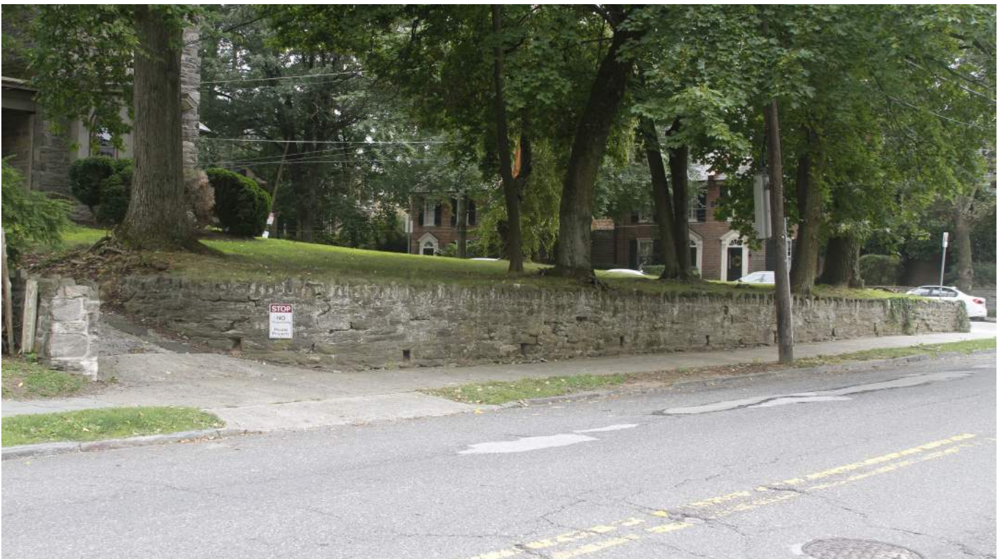
6. Schist retaining wall, looking south from E. Chestnut Hill Ave.
