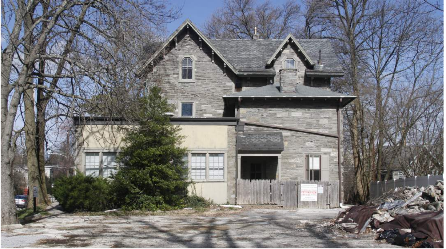
5. Southeast elevation, looking northwest from rear of parcel.
