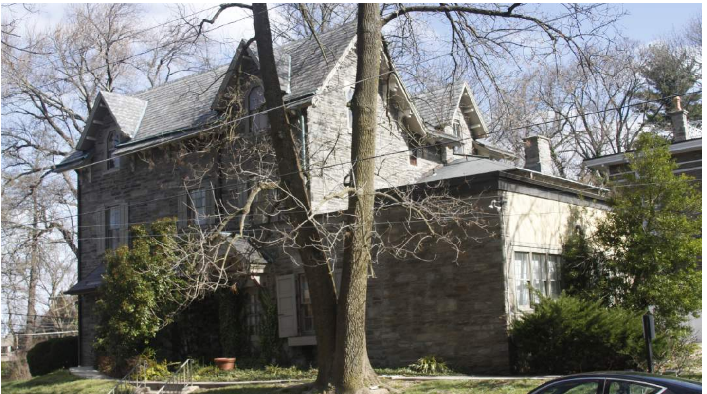
4. Southwest and southeast elevations, looking north from Germantown Ave.
