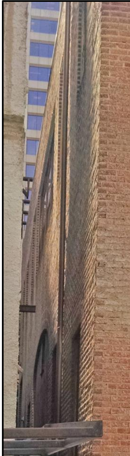
North/rear elevation with limited visibility. Source: J.M. Duffin.
