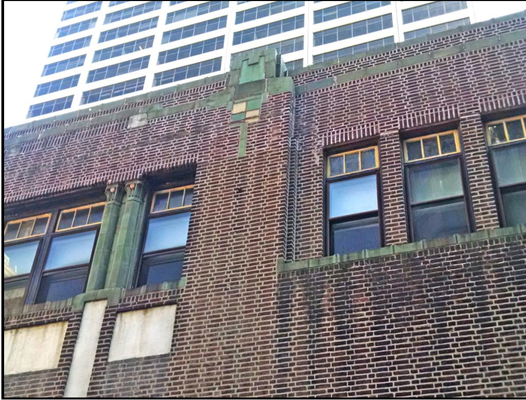
Upper floor details of the front facade. Source: J.M. Duffin.
