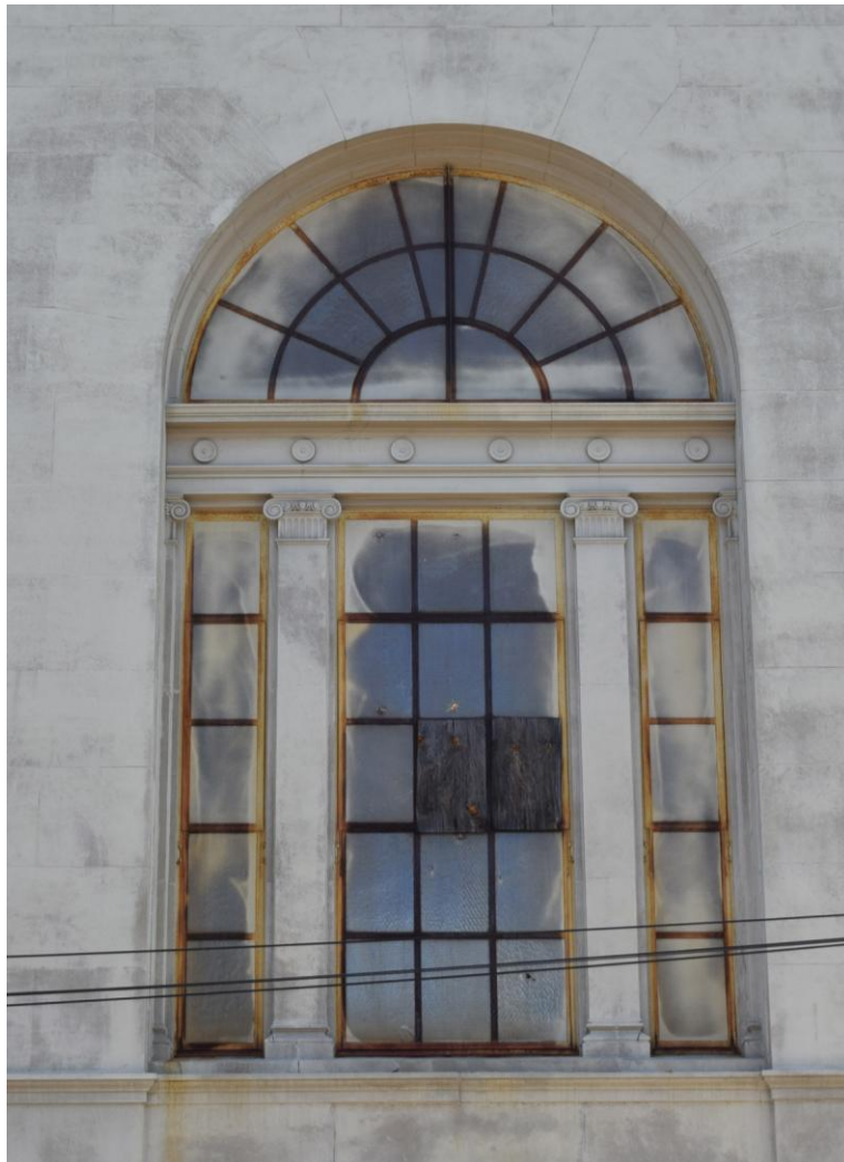
Figure 8: Window detail (façade). Photograph by author, August 2017.
