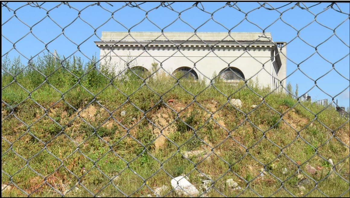
Figure 10: Jasper Street view of the eastern elevation previously obscured by the Bromley Mill. Photograph by author, August 2017.
