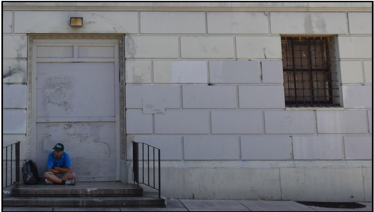
Figure 4: Door surround and window grill. Photograph by author, August 2017.
