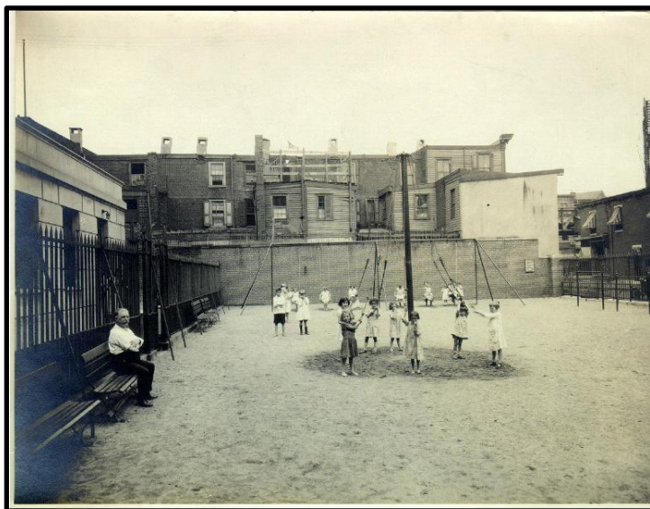
Figure 16: Playground at the Western's Front & York office, looking west. The extension facing Boston Street is visible at the left.
