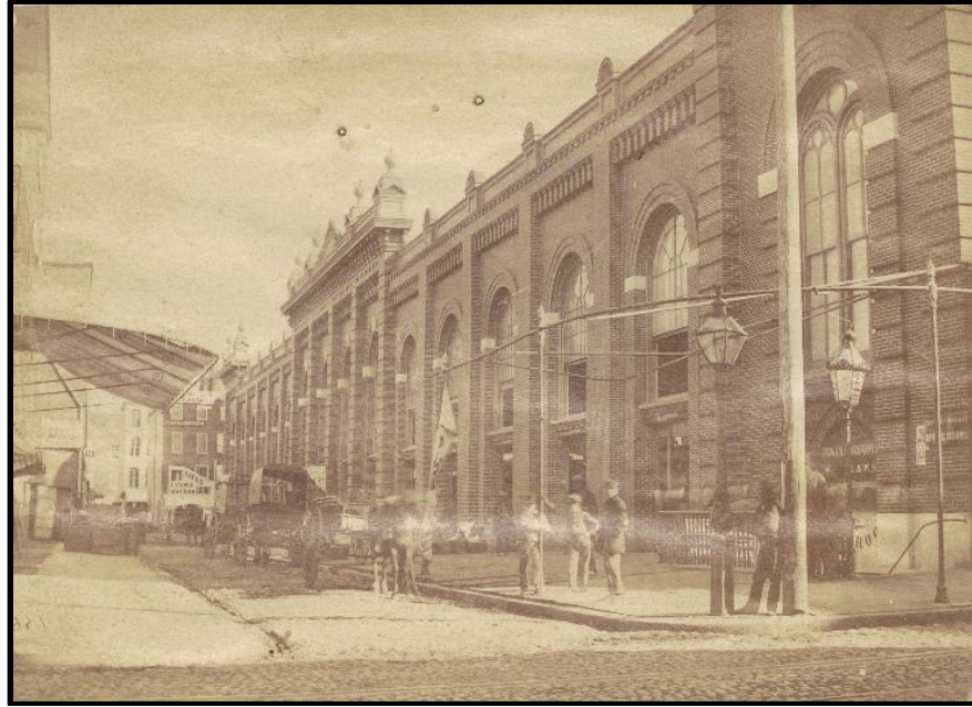
The “Fifth St. Market,” more formally known as the Eastern Market House at Fifth and Merchant Streets, as it appeared in the 1860s. Source: the Castner Collection, the Free Library of Philadelphia.
