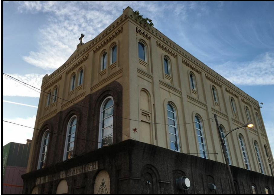
Looking southeast at the primary and east elevations. Source: Oscar Beisert.
