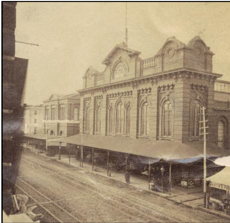
The Farmers Market House at 12 th and Market Streets. Source: the Castner Collection, the Free Library of Philadelphia.
