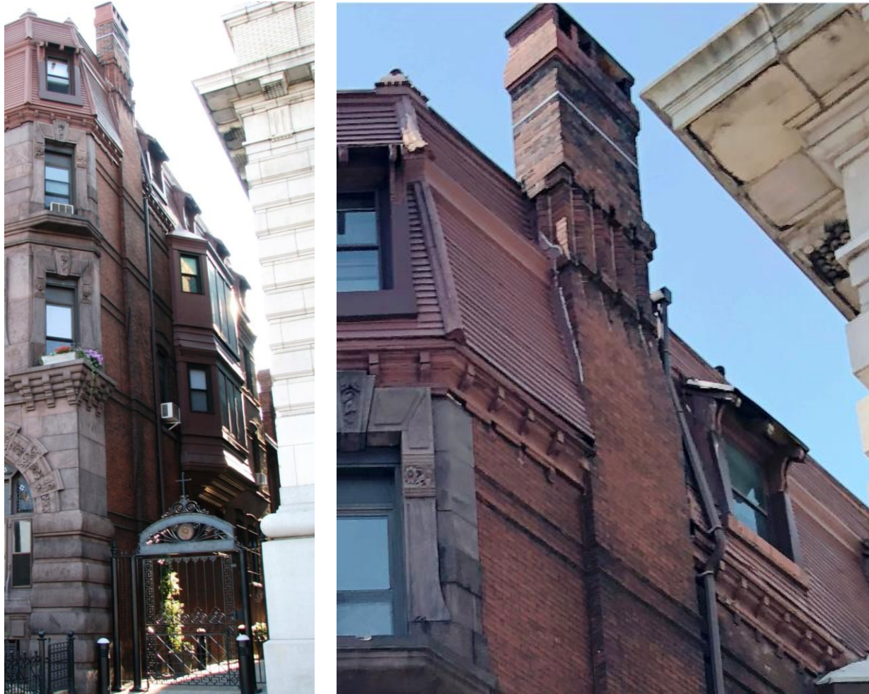
Figure 9: The north elevation faces St. Rita's Church and is visible from the public right-of-way along a nine-foot wide passageway between the buildings. Character-defining features of the façade include decorative brickwork, three-sided metal bay window, elaborate brick chimney, ribbed metal mansard roof, and shed dormer windows.
