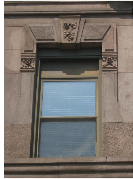
Figure 7: Details of the upper floors of the front façade. The windows in the top floor and second floor have been replaced. The second floor windows have been slightly built down within the original masonry opening.
