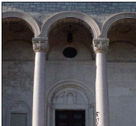
Fig. 18. Detail of south entry loggia.
