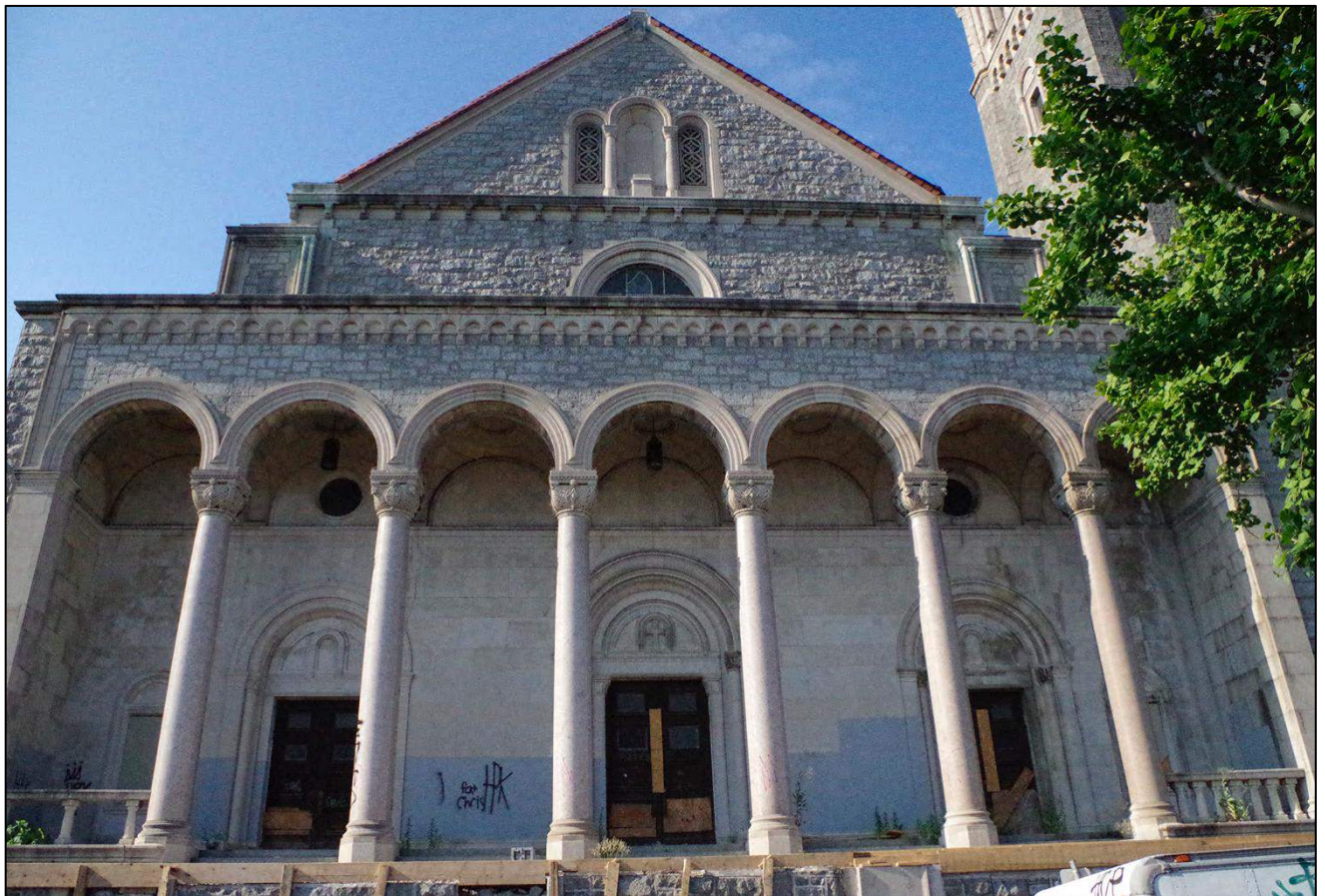
Fig. 3. South elevation with colonnade and entry loggia.
