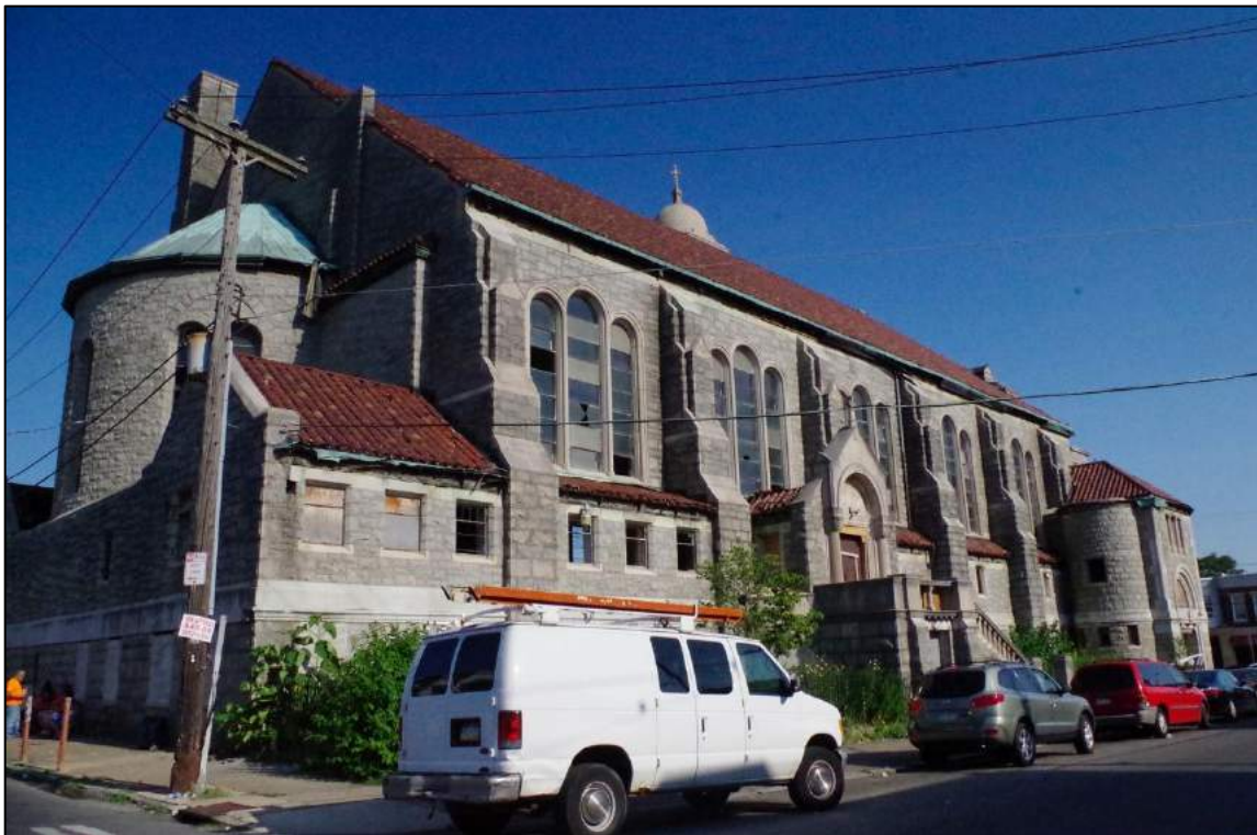
Fig. 7. View of the northwest corner of the church.
