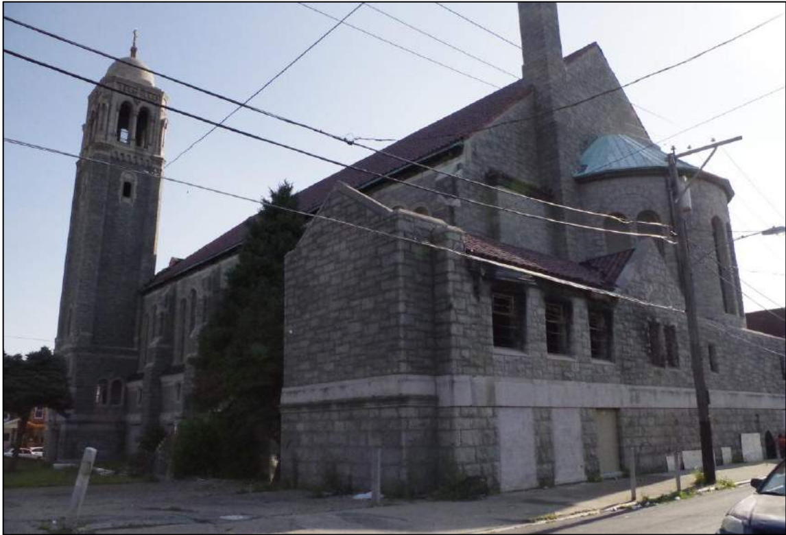
Fig. 10. View of the church from the northeast.
