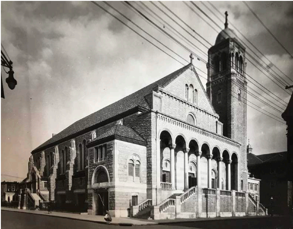
Fig. 23. An "as-built" photograph of Ascension of Our Lord Church in 1928. William Rittase, photographer. Source: Athenaeum of Philadelphia, Hoffman-Henon Collection.
