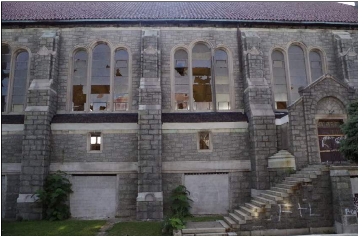
Fig. 11. East elevation of the church showing missing window panes and a staircase without its balustrade.
