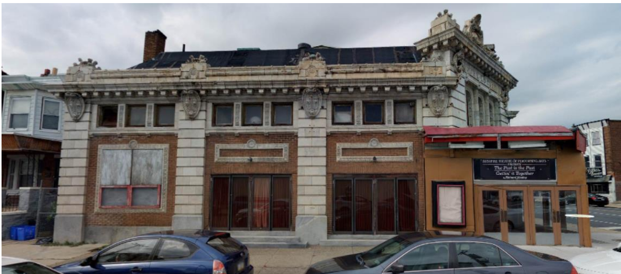
South elevation along Locust Street. Source: Cyclomedia, July 2017.
