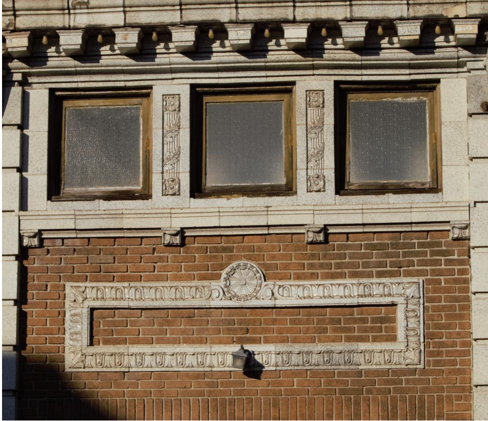
Figure 5. A detail of one of the Locust's bays featuring the waterleaf banding and row of windows common to all seven bays.
