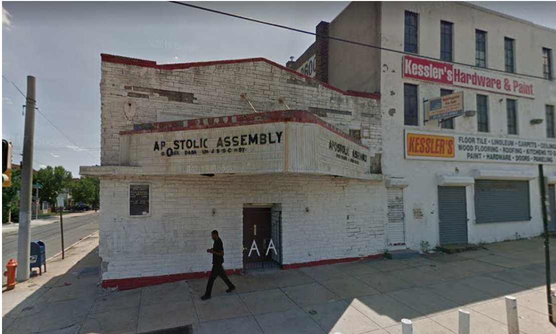
Figure 28. The former Strand Theatre, now clad in formstone, 1200-02 W. Girard Avenue. Source: “Bushfire,” Cinema Treasures .
