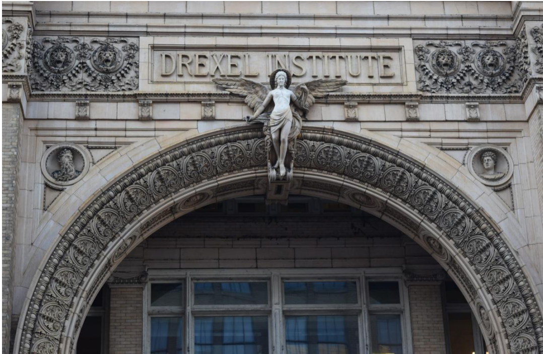
Figure 25. The elaborate entry of the Drexel Institute, done in Conkling-Armstrong terra cotta. Source: Author, 2017.
