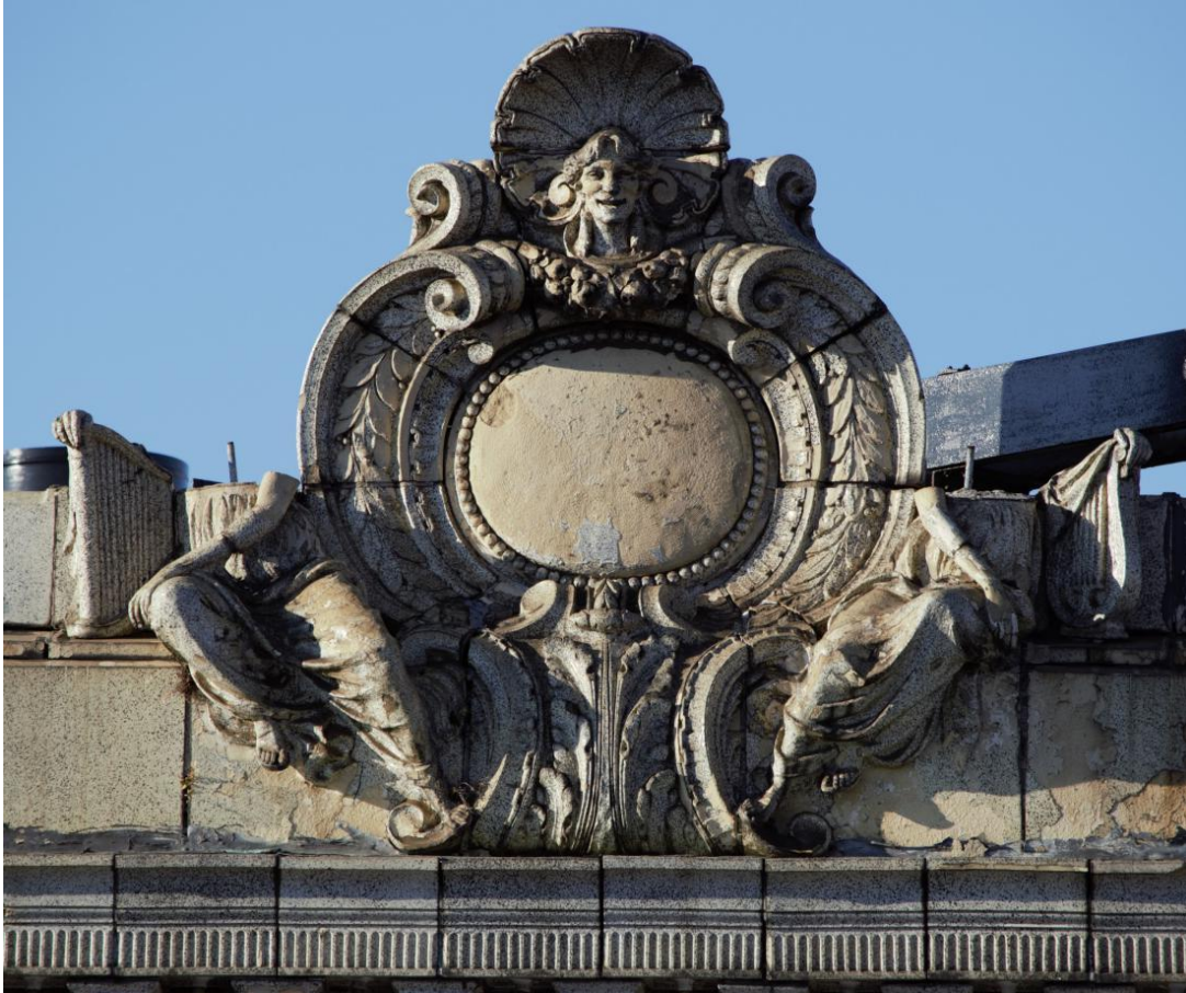
Figure 12. Detail of the Locust's central cartouche as it appears today with the flanking figures incomplete. Compare with Figure 13.
