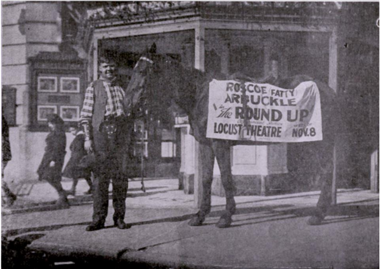
Figure 14. A publicity stunt outside the Locust advertising the movie Round Up in 1920. The original marquee is visible in the background. Source: “Bushfire Theatre,” Cinema Treasures , accessed December 21, 2017. http://cinematreasures.org/theaters/3450/photos .
