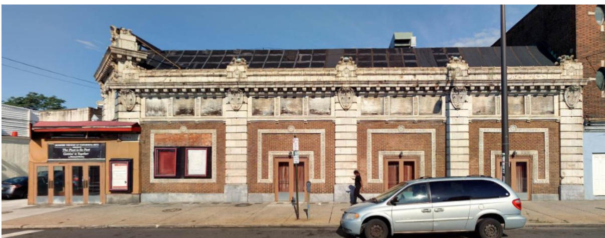
East elevation along S 52 nd Street. Source: Cyclomedia, July 2017.
