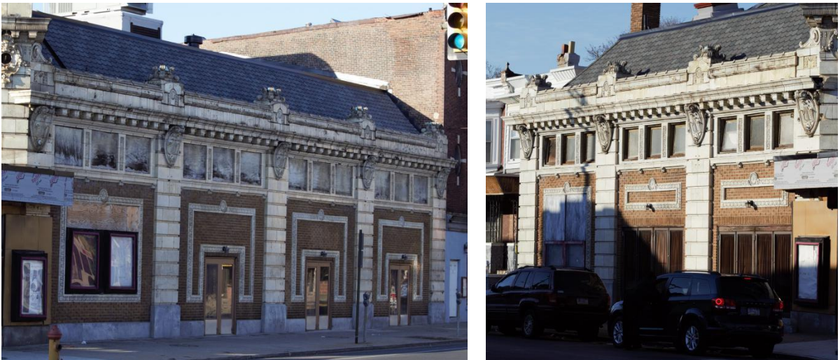
Figure 4. The west and south facing facades of the Locust, featuring seven bays separated by rusticated piers.
