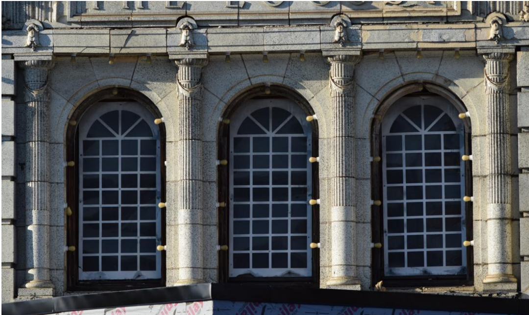
Figure 9. The arched windows of the Locust's chamfered entry facade, flanked by Doric pilasters and studded with light bulbs.
