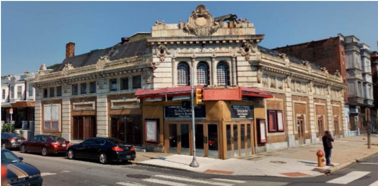
Southeast corner. View from intersection of S 52 nd and Locust Street. Source: Cyclomedia, July 2017.
