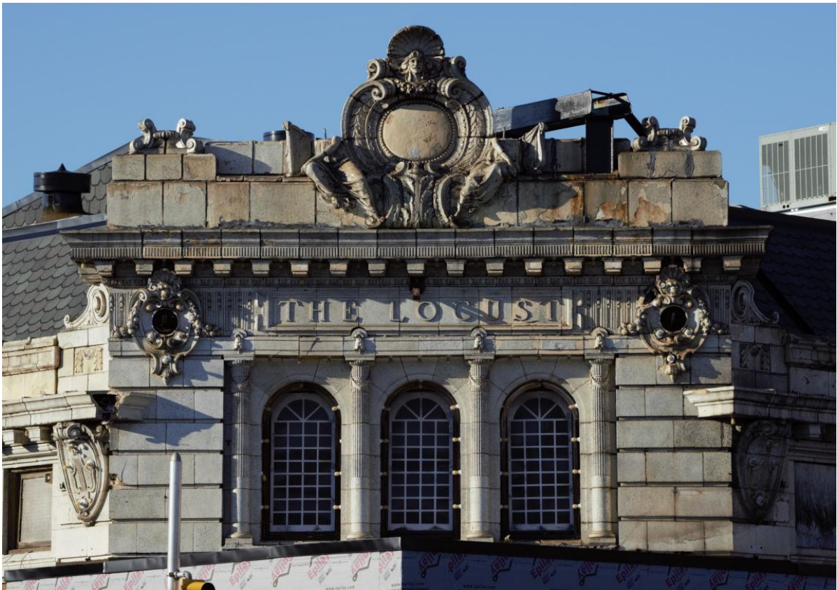
Figure 8. The Locust’s chamfered front entry done entirely in terra cotta.
