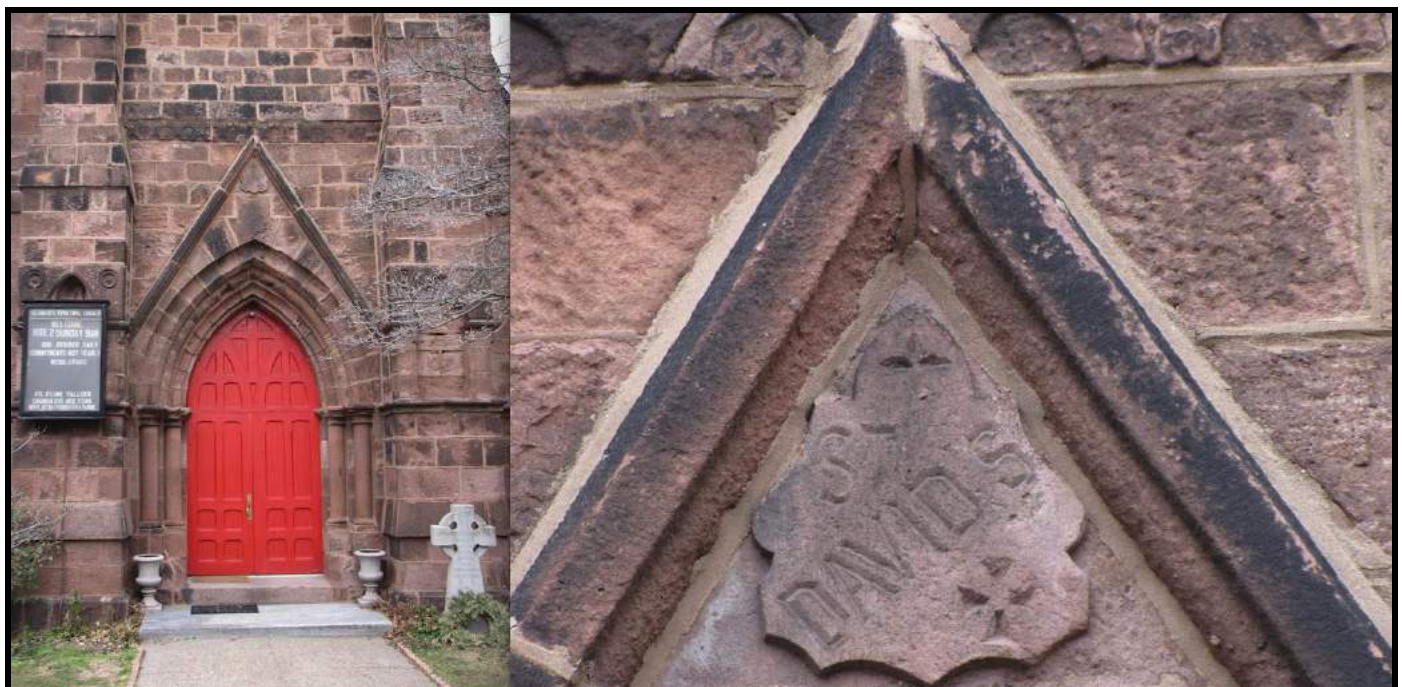
Bottom of Tower: South façade at the front door.
