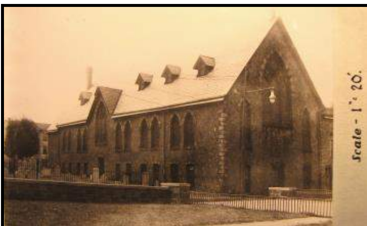
PHOTO: EAST FAÇADE AND REAR OF THE BUILDING - MUTUAL INSURANCE POLICY OF 1947 – ACCESSED AT HSP - 15 TH SEPTEMBER 2017 BY J. J. MENKEVICH
