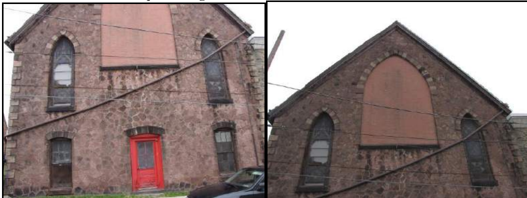
This Building fronts on Kram Avenue.
