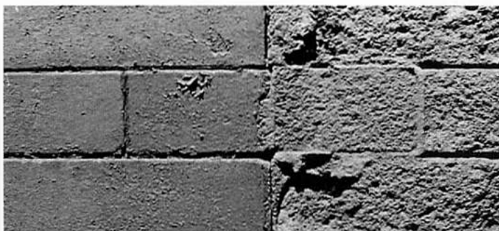
The negative effects of abrasive cleaning or sandblasting on brick are evident on the right.
