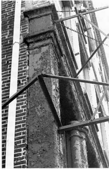
Deteriorated cast iron.
