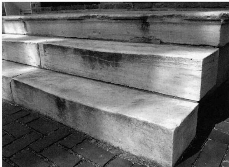
Masonry steps should be maintained to prevent the damaging effects of water penetration.
