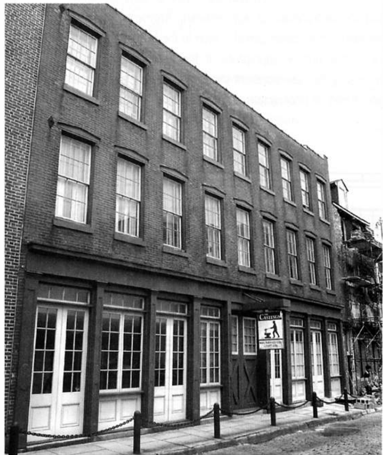
Thin wood muntins and decorative cornices are typical storefront details.
