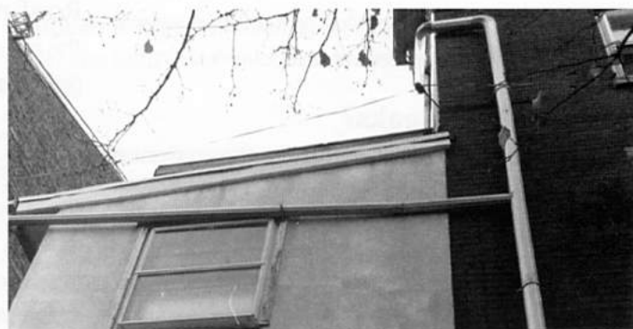
An inappropriate gutter treatment.
