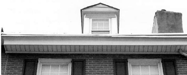
Aluminum cladding hides the original cornice details.
