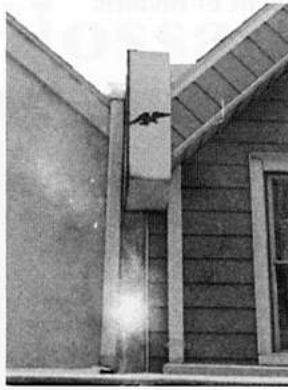
Inappropriate gutter treatment
