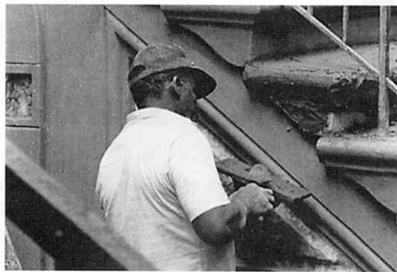
A mason applying a finish coat of stucco.
