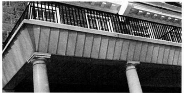
Aluminum cladding hides the original cornice details
