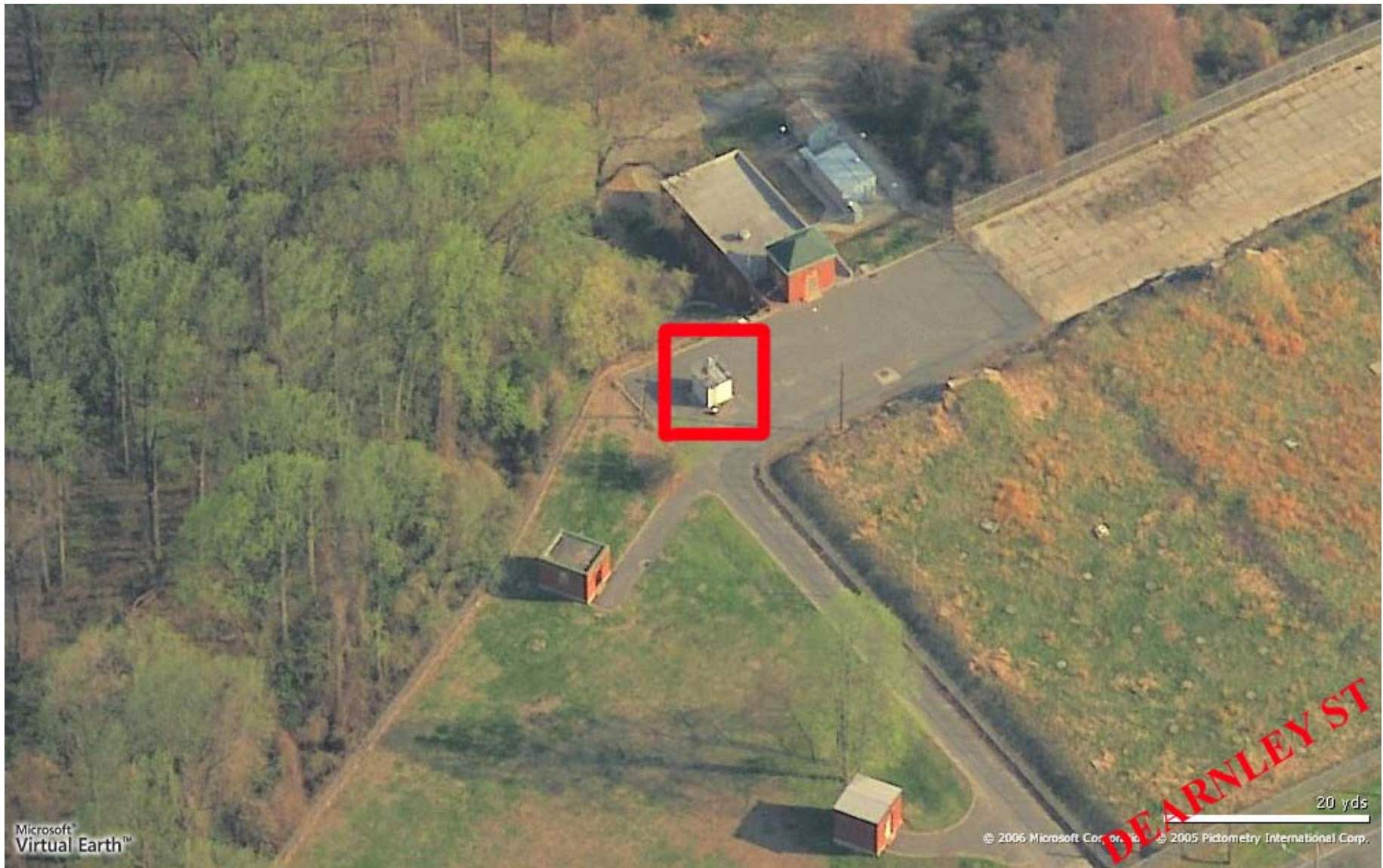
Figure 5 – ROX North Aerial View
