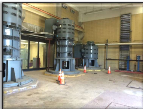
Figure 22: Effluent Pump Station Prior to Installation of Sixth Pump
