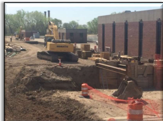
Figure 18: Ongoing Construction of Two Bypass Conduits to Expand Wet Weather Handling Capacity of Northeast WPCP
