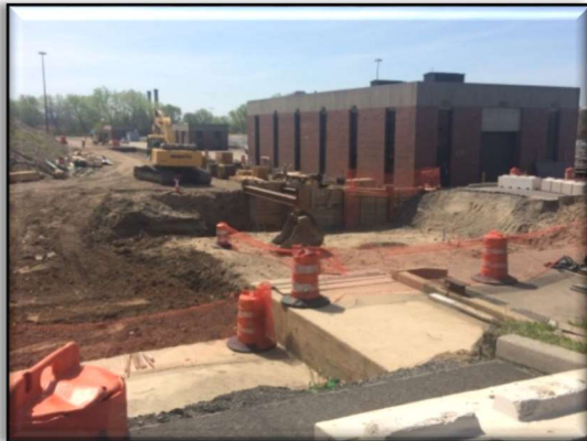
Figure 18: Ongoing Construction of Two Bypass Conduits to Expand Wet Weather Handling Capacity of Northeast WPCP
