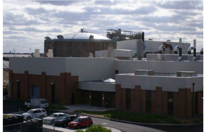
The Northeast WPCP biogas cogeneration facility (Photo: PWD staff).
