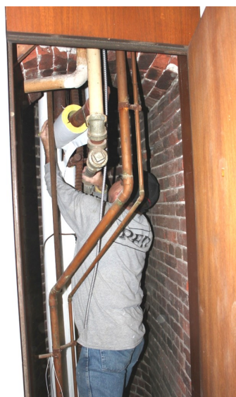
Pipe Insulation Installation
