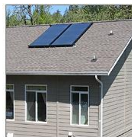
Figure 2-1: Solar Water Heating System Source: U.S. Department of Energy
