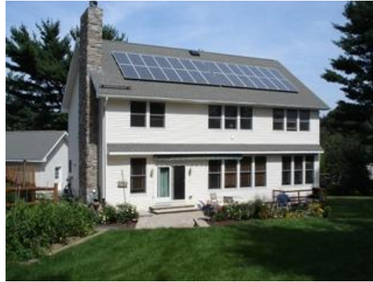
Bradley 5.12 kW PV System, Philadelphia
