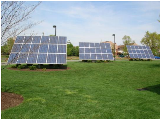
Figure 2-10: Ground Mounted PV System (Three Eagles-Nova Care)
