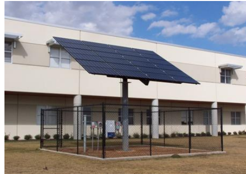
Figure 2-12: Pole-mounted PV system for a Middle School
