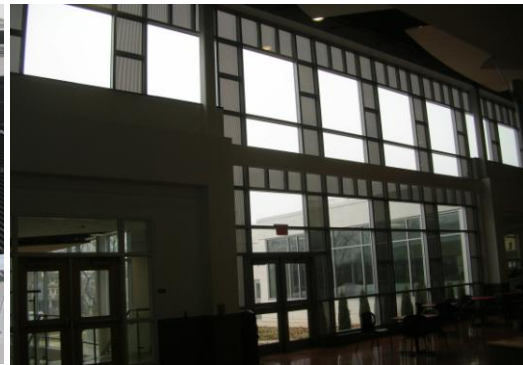
Figure 2-6: PV Modules allowing light to filter through interior windows, Microsoft School, Philadelphia
