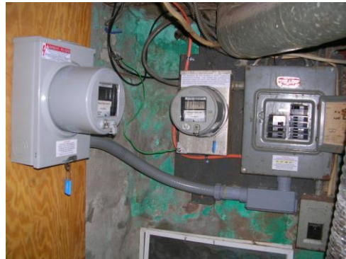
Figure 4-1: PECO Meters (OUT – left; IN – right) Row Home; Northern Liberties, Philadelphia
