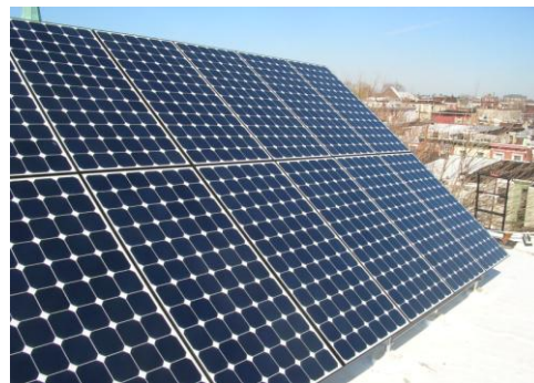
2.94 kW Rooftop PV System, Philadelphia
