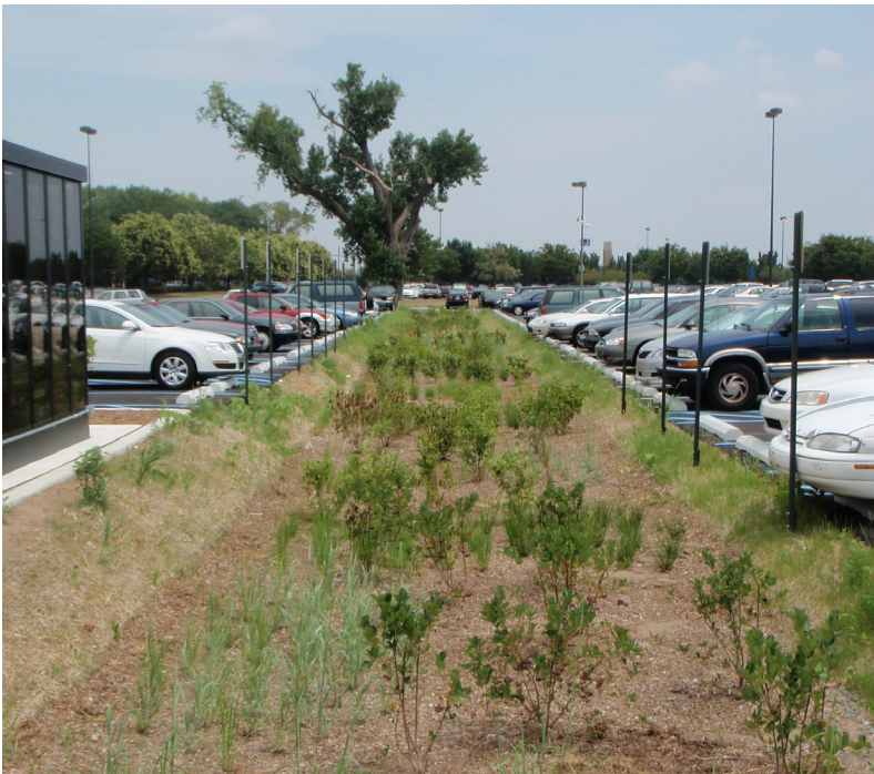
Above: A vegetated swale collects and infiltrates stormwater from an employee parking lot at the Philadelphia International Airport in the Schuylkill Watershed.
