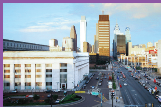
30th Street Station looking east on Market Street (Source: Station Square Urban Design Study, 2008)
