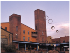
Sherman Mills, adaptive reuse
