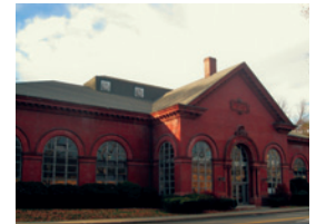
Belmont Pumping Station
