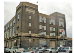
Reed Street Radio and Fleet Maintenance
