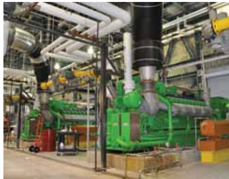
PWD's 5.6 MW Biogas Cogeneration Plant went into service in November 2013.
