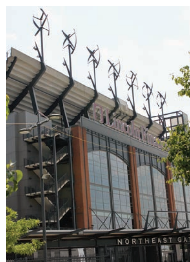
Vertical axis wind turbines at Lincoln Financial Field.
