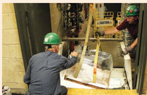
Workers install a new boiler as part of the City's guaranteed energy savings project.
