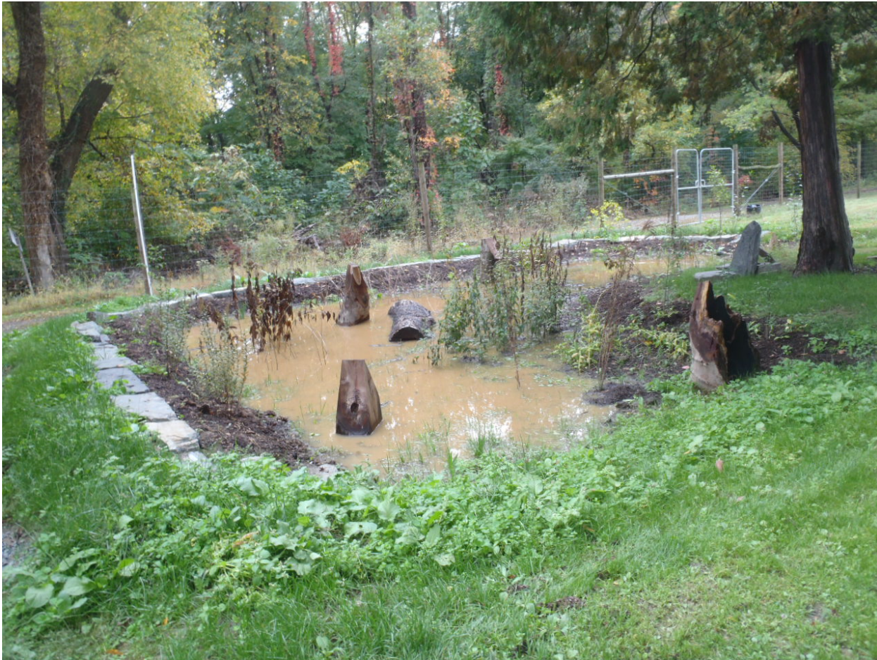
The newly installed rain garden at Greenland Nursery was put into service during the mid-October rainstorms.
