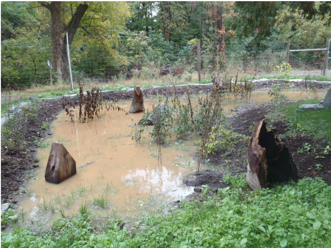
Stormwater runoff from the nursery structures and driveway is now diverted into the rain garden basin.
